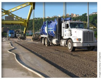
Hydrodemolition permits removal of bridge deck concrete more quickly and safely than traditional mechanical methods and can address both moderate and severe deck deterioration.
