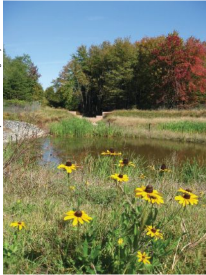
An extended detention pond in Anne Arundel County, Maryland.
