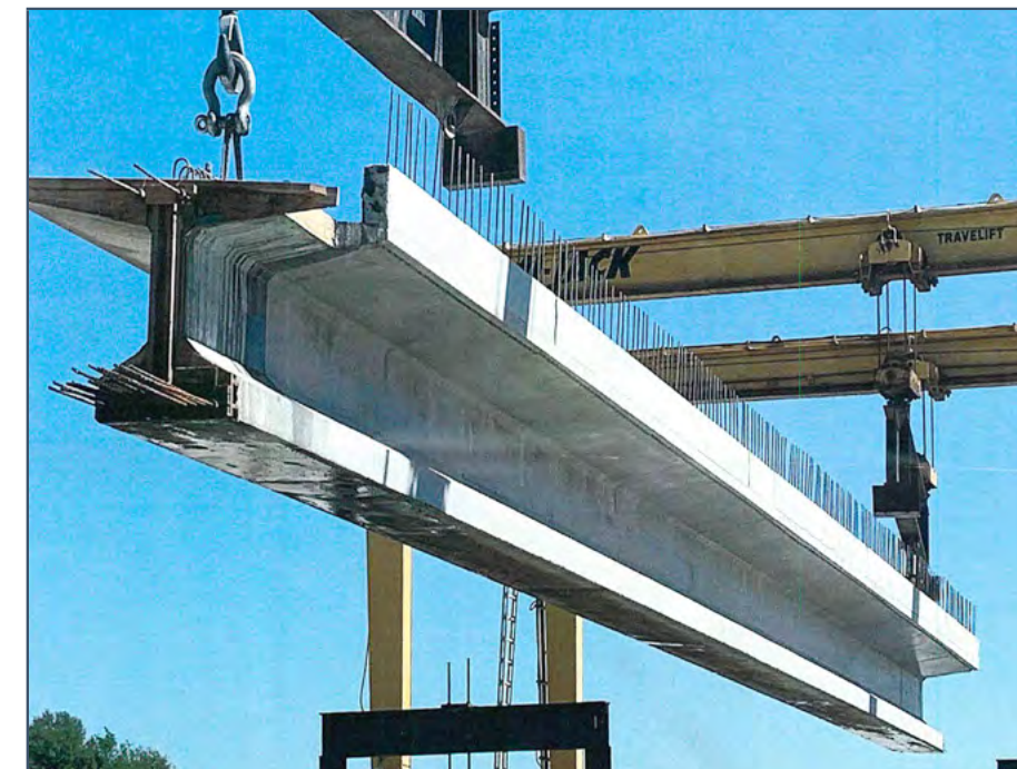
Figure 24. Girder prefabricated with a partial-depth deck overhang from Texas DOT
