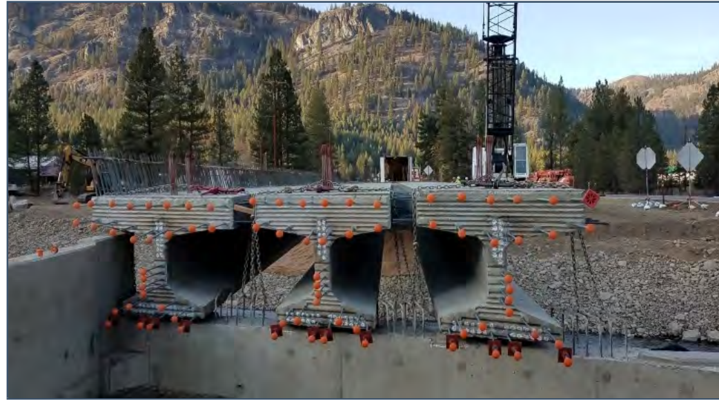
Figure 25. Decked bulb tee girders from Washington DOT
