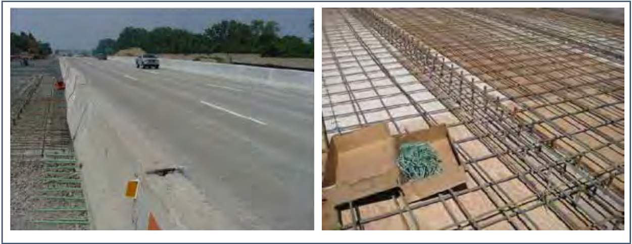
Figure 18. Bridge deck with ASTM A1035 bars built in 2003 in Michigan (left) and in 2008 in Utah (right)
