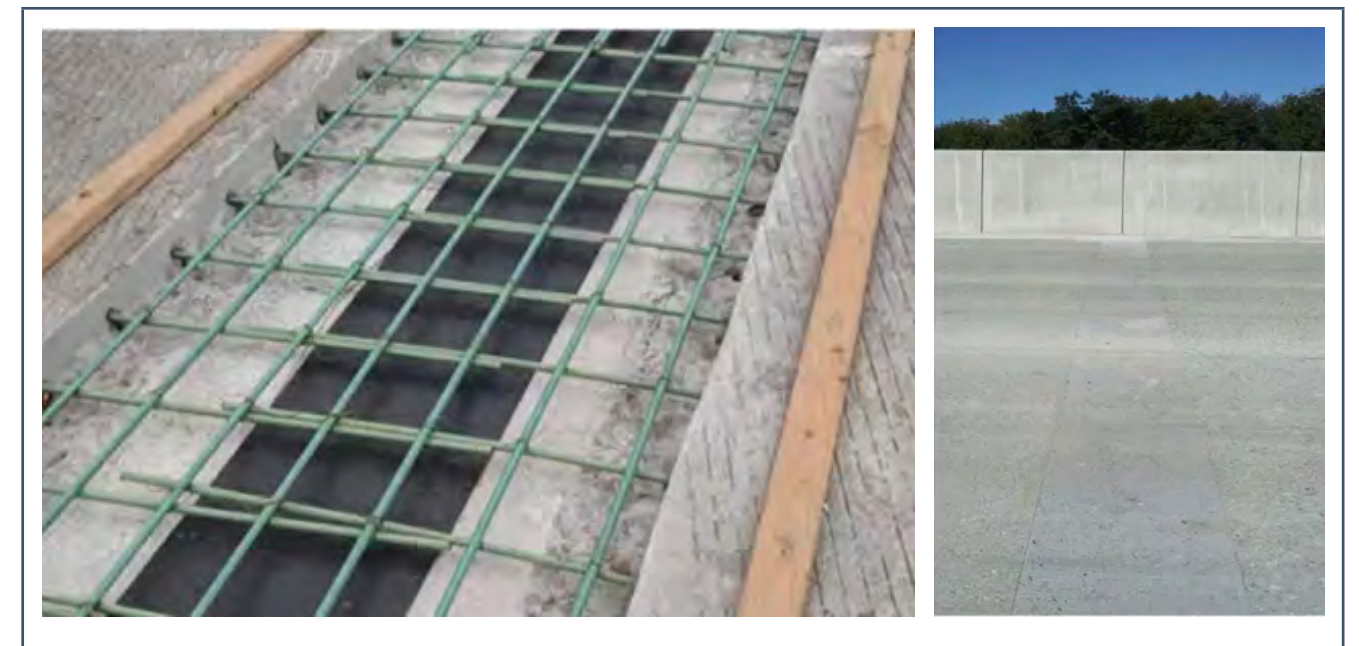
Figure 7. Link slab construction (left), finished link slab (right) from New York State DOT
