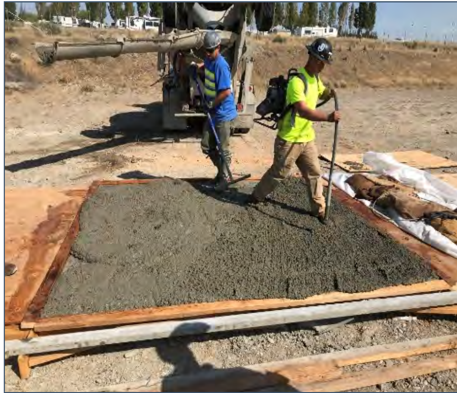
Figure 31. A 10 ft. by 10 ft. test pour by Washington DOT
