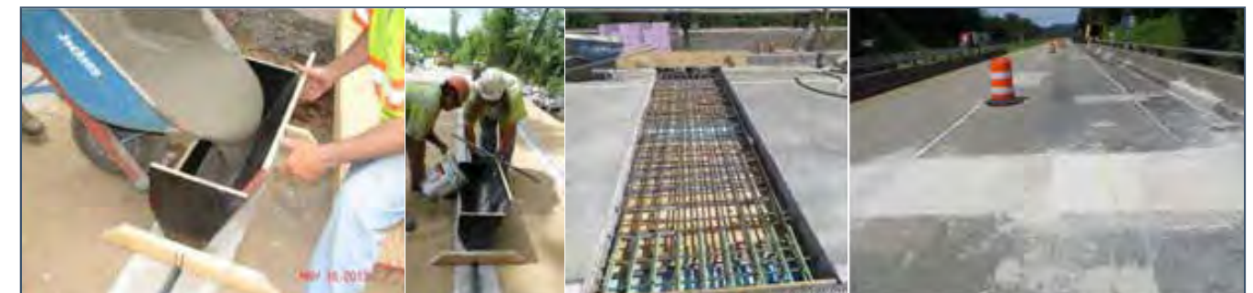
Figure 5. A fiber-reinforced Engineered Cementitious Composite (ECC) mix used for a shear key (left), fiber-reinforced concrete used for a link slab (right) in Virginia
