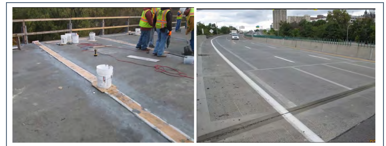
Figure 10. Sealing of precast deck panel forms for UHPC joints (left), finished joints (right) from New York State
