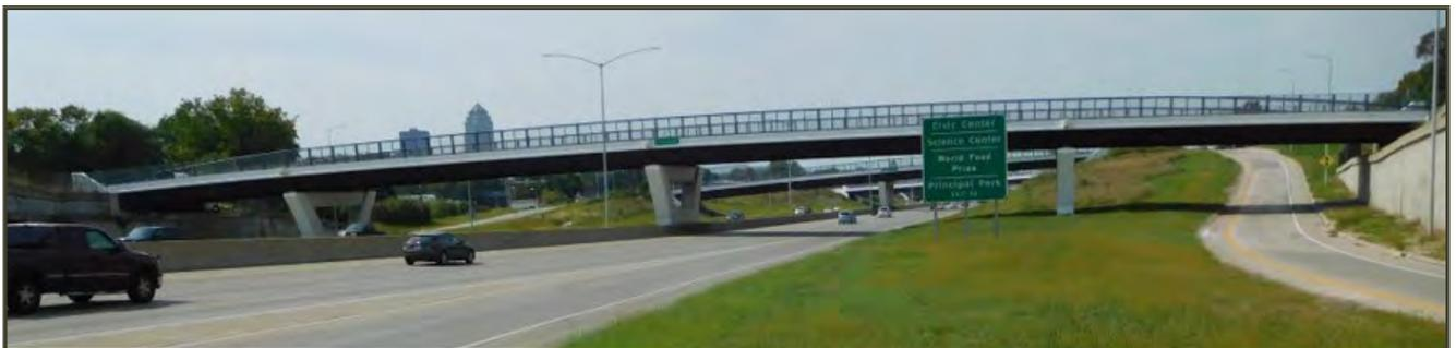
*Figure 3 Iowa 426 foot long Continuous Welded Steel Girder*
