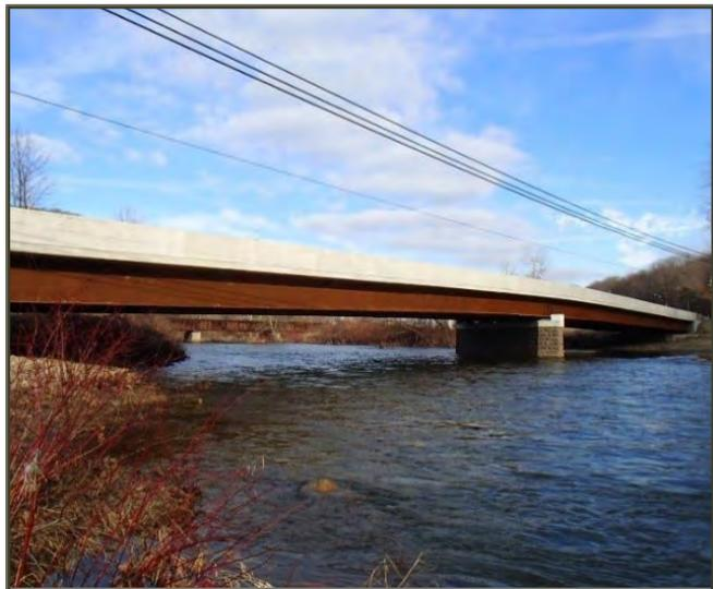
*Figure 8 PennDOT 373 foot. Steel Jointless Bridge*
