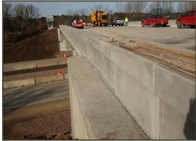
*Figure 7 MnDOT Semi-Integral Abutment with Barrier on top of Approach Panel*
