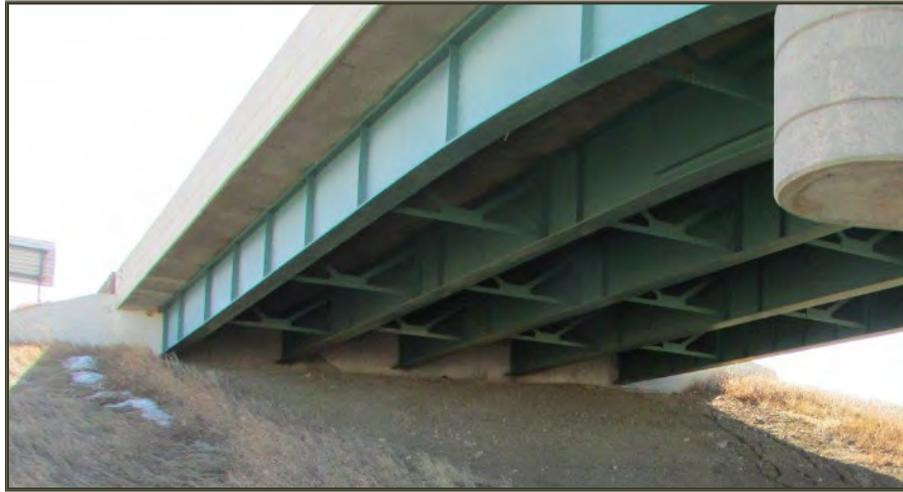
*Figure 9 SDDOT Steel Girder Bridge with Integral Abutment*
