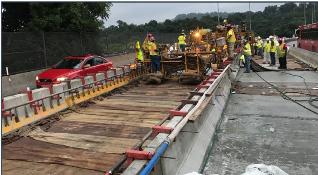
**Figure A-4 Example of an LMC placement operation: placing curing covers behind finishing operation (Pennsylvania DOT)**
