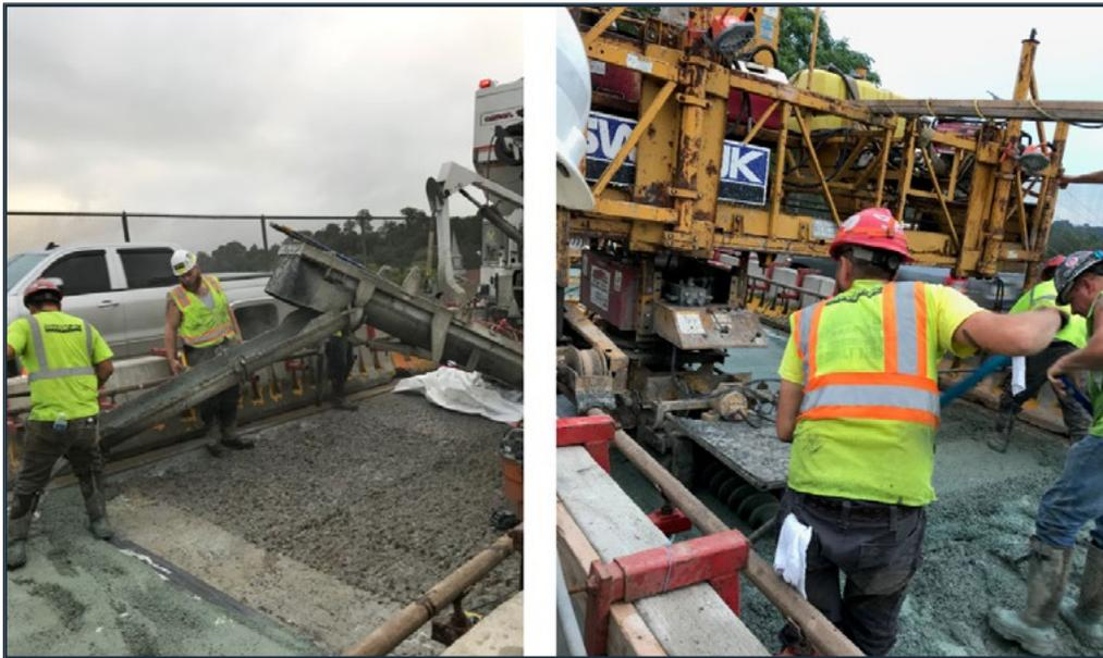
**Figure A-3 Example of LMC placed with LMC mixer truck and finished with Bid-Well finishing machine (Pennsylvania DOT)**
