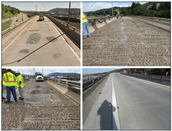
Figure A-6 SR8029 project (left to right, top to bottom): a) before preservation project, b) and c) after scarification and hydrodemolition, and d) after LMC overlay (Pennsylvania DOT)
