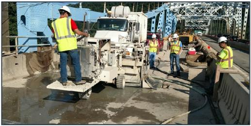
Figure A-2 Example of hydrodemolition machine calibration (Pennsylvania DOT)
