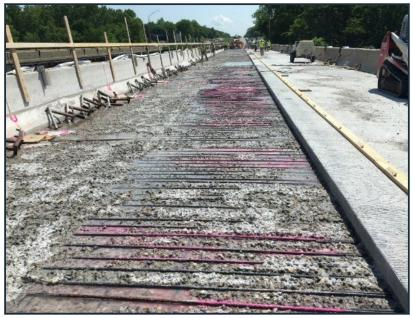
Figure A-13 Marked reinforcing steel showing bars that have unbonded with surrounding concrete (Michigan DOT)
