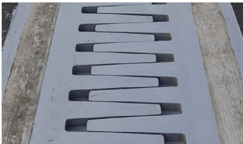
*Figure 2.4-38. Steel Finger Joint*
