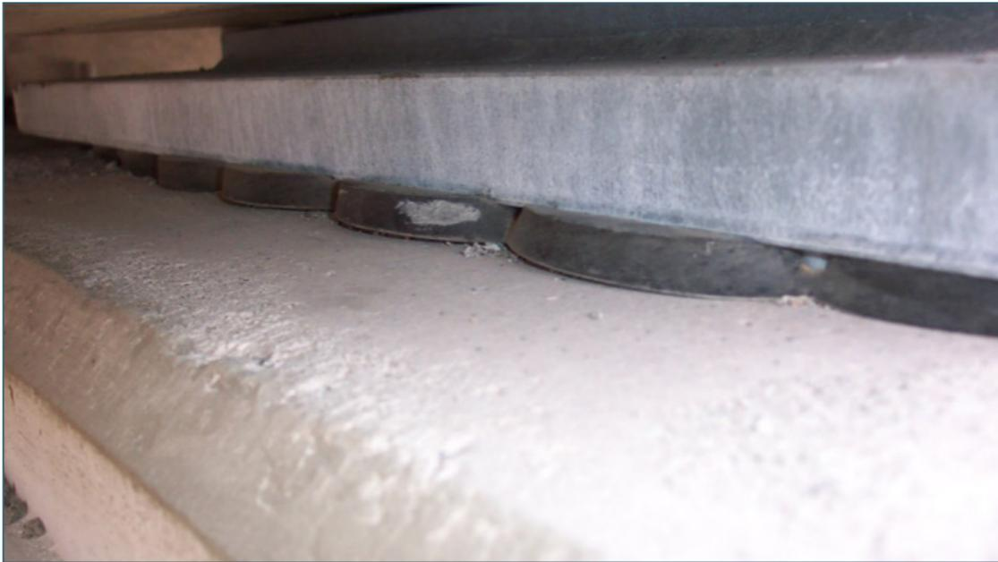
*Figure 2.3-18. Plain elastomeric pad squeezing out from under masonry plate (MN)*
