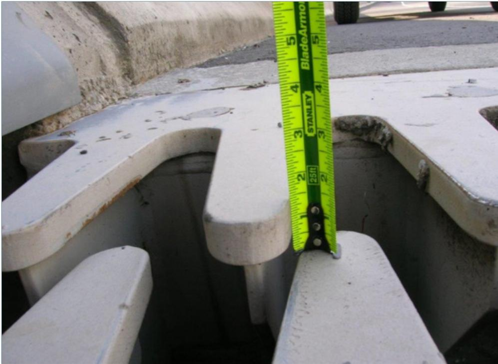
*Figure 2.4-40. Finger Joint: vertical displacement due to girder twist.
