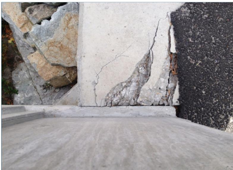
**Figure 2.4-9. Concrete cracked by failure to account properly for movements. (NY)**
