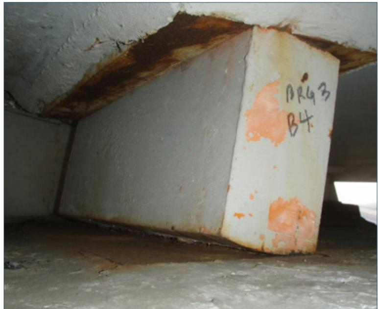
**Figure 2.3-5. Single roller bearing (OR)**
