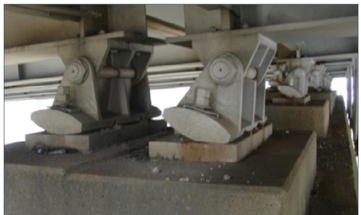
**Figure 2.3-9. High movable rocker bearings. (LA)**
