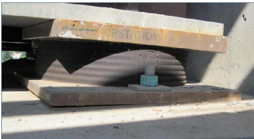
**Figure 2.3-16. Over-rotation, possibly due to initial camber. Note uplift at front edge and bulging at back. (NY)**
