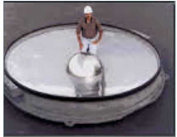
**Figure 2.3-27. Friction Pendulum Bearing for the Benicia-Martinez Bridge (EPS)**
