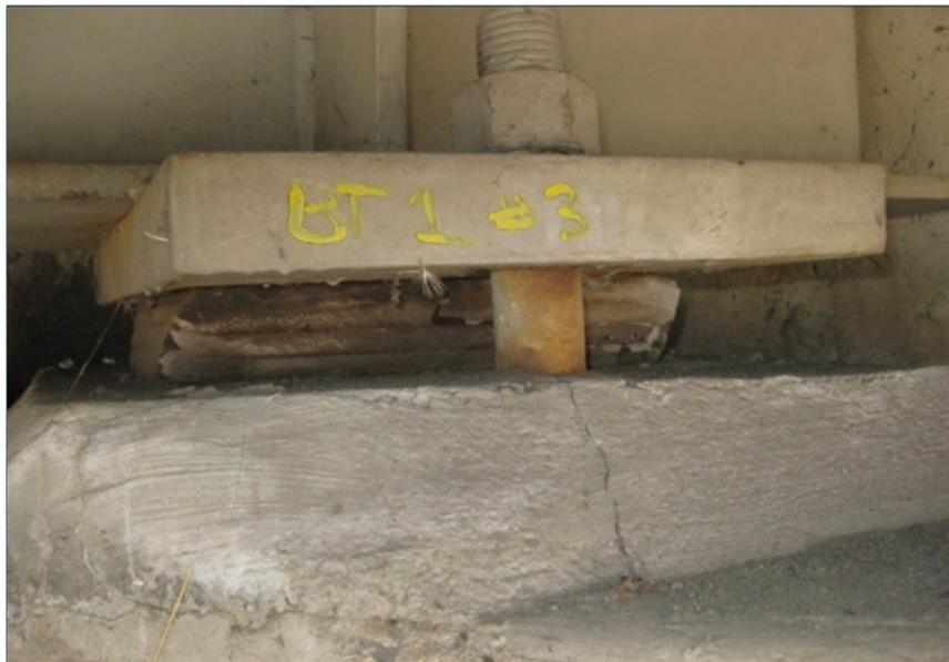
*Figure 2.3-33. Steel reinforced elastomeric bearing - cracked grout pad*
