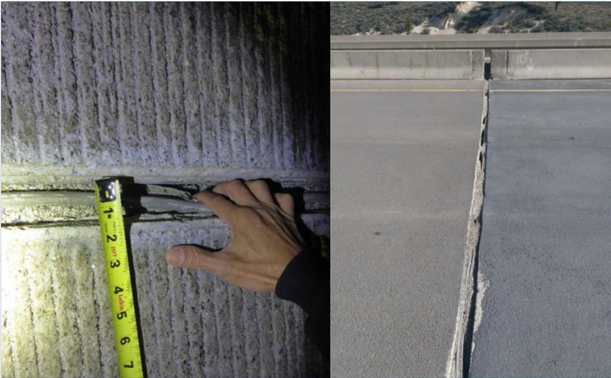
Figure 2.4-31. Adhesive-bonded strip seal failure.
