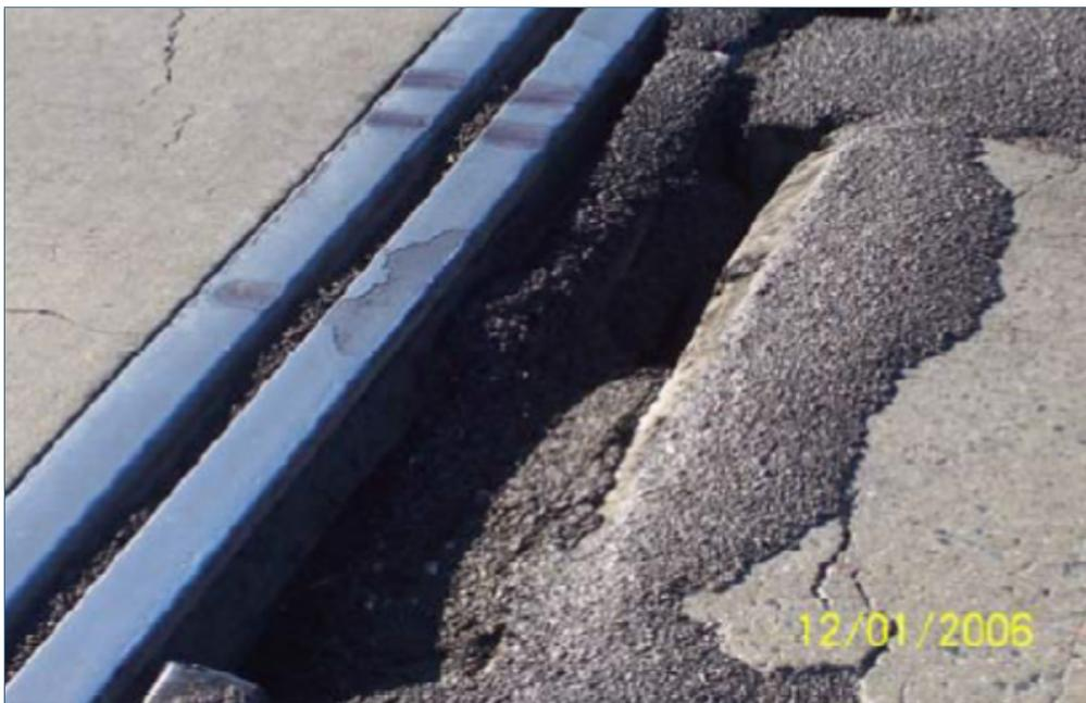
*Figure 2.4-43. Modular Joint: header failure (CA)*
