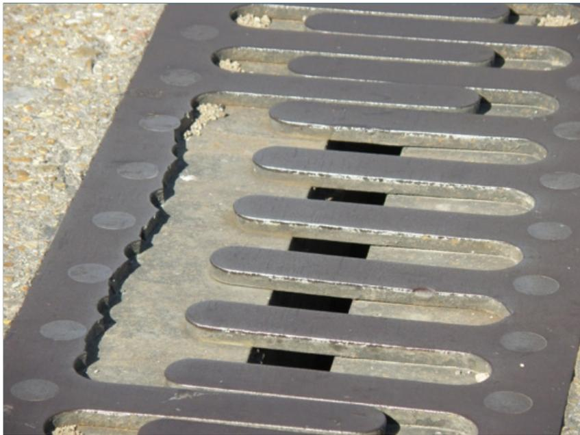
**Figure 2.4-39. Finger Joint: Fractured fingers (LA).**
