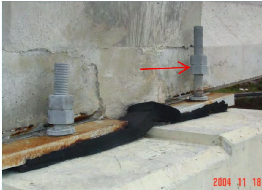
*Figure 2.3-31. Elastomeric bearing set on epoxy base and squeezing out*
