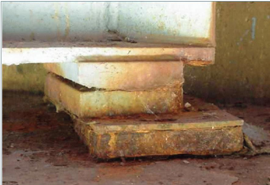
*Figure 2.3-12. Low rocker (with sliding plate under)*
