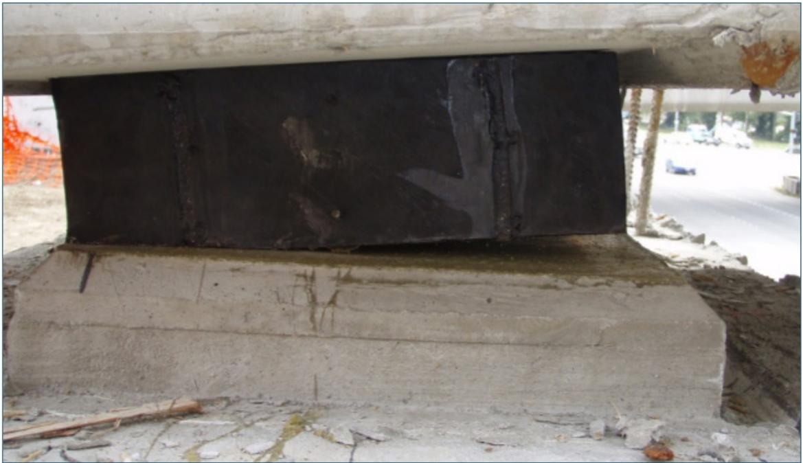
*Figure 2.3-2. Girder with reversed bearing recess*
