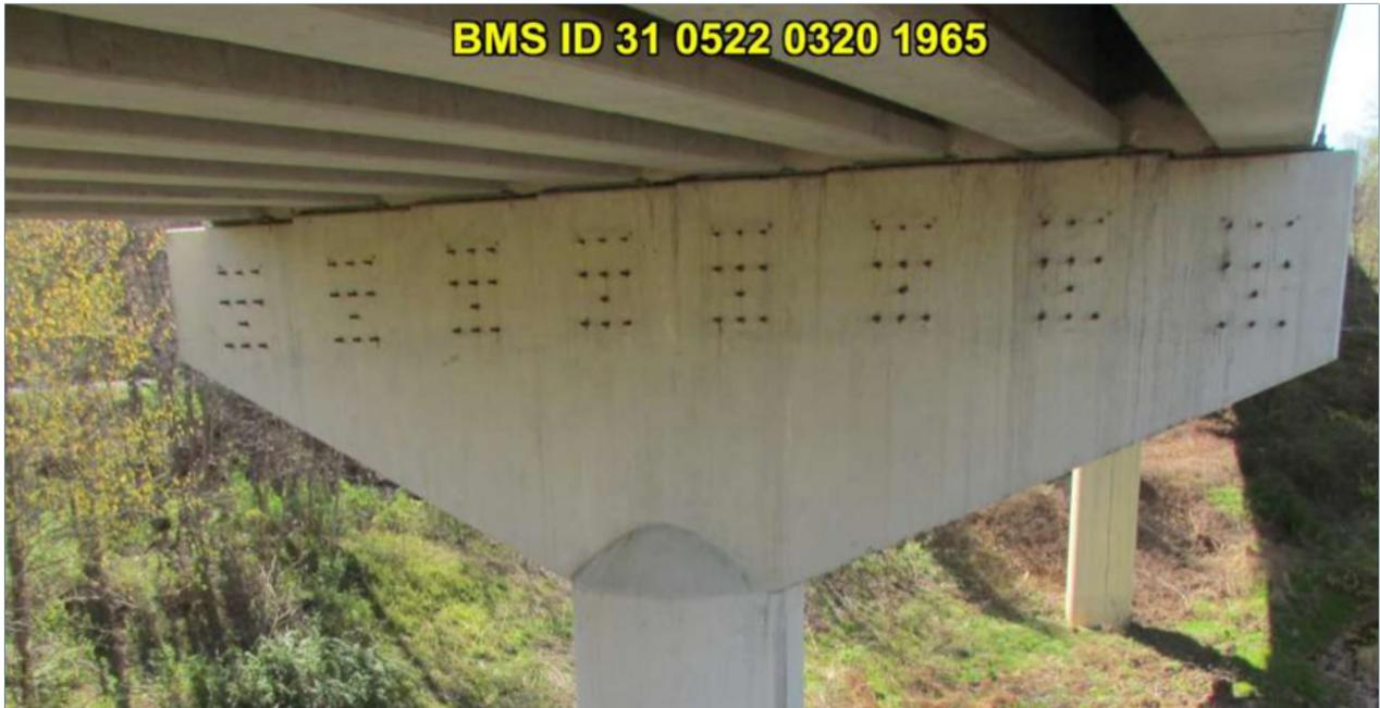
*Figure 2.3-36. Provision for bolted lifting bracket (PA)*
