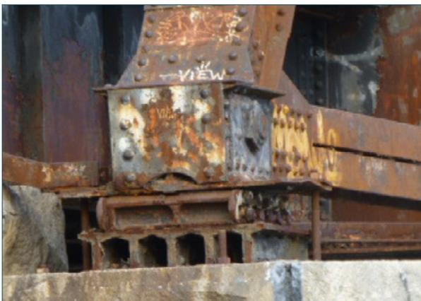
**Figure 2.3-8. Roller nest showing corrosion (CA)**
