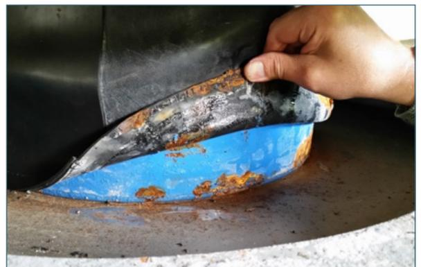
**Figure 2.3-28. Corroded isolation bearing (WA)**
