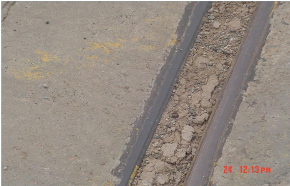
Figure 2.4-46. Debris in joint
