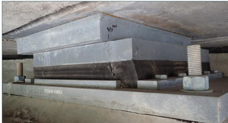
*Figure 2.3-41. Bolted stopper plates for elastomeric bearings*
