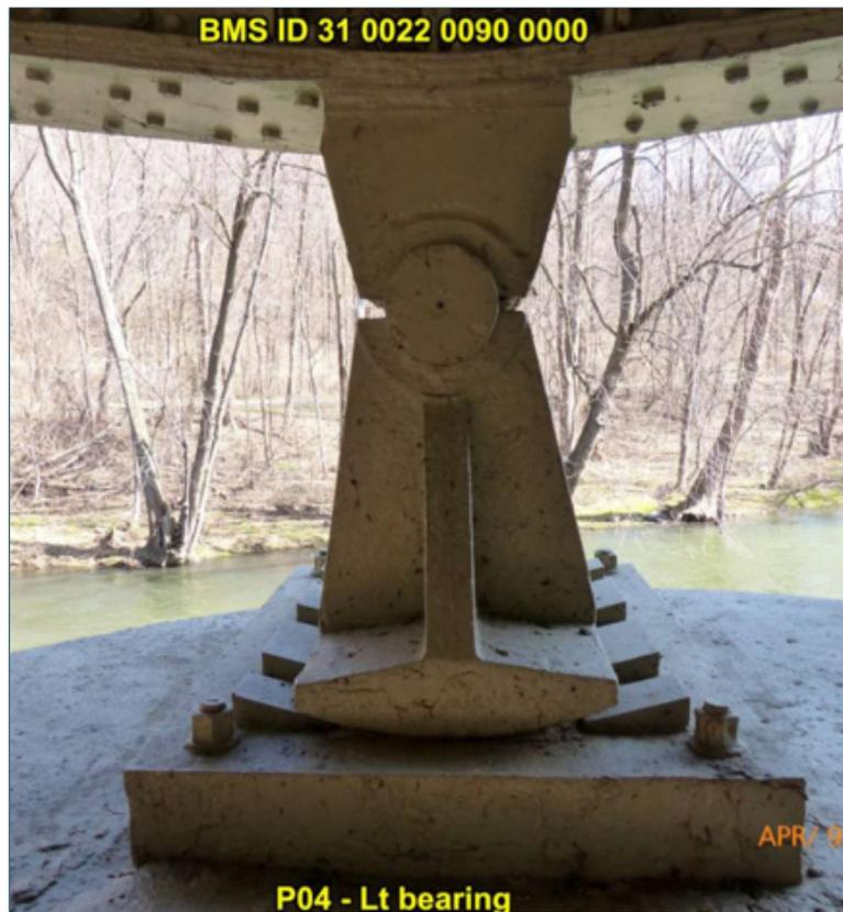
*Figure 2.3-39. Keeper plate retrofit for rocker bearing (PA)*
