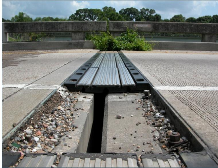
*Figure 2.4-33. Bolt-down elastomeric panel, showing failed bolts. (LA)*
