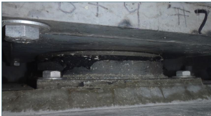
*Figure 2.3-21. Elastomer leaking from pot bearing (OR)*
