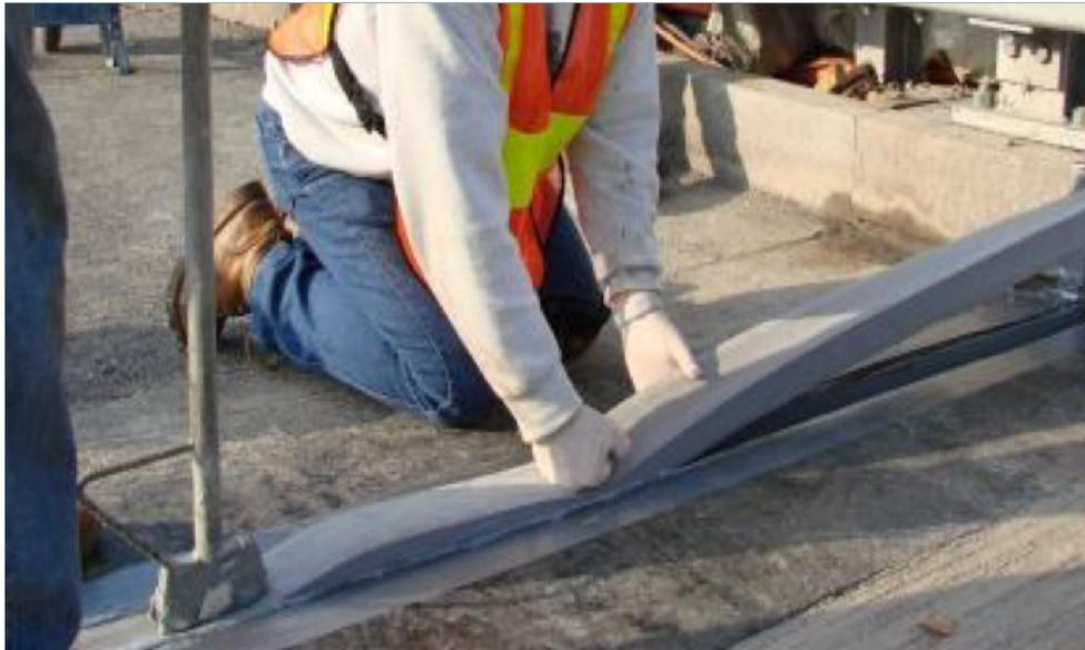
*Figure 2.4-25. Installation of foam joint*
