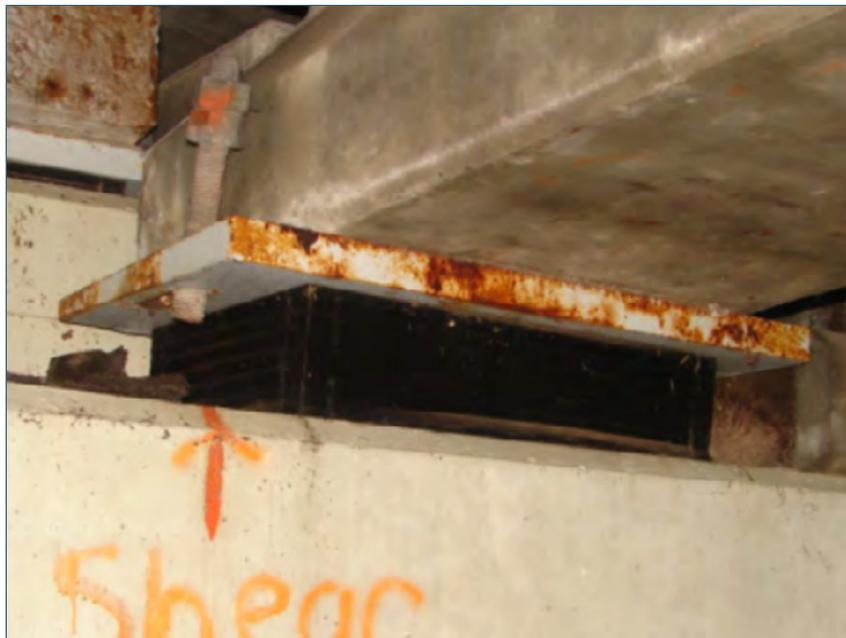
*Figure 2.3-32. Steel reinforced elastomeric bearing - broken anchor bolt*
