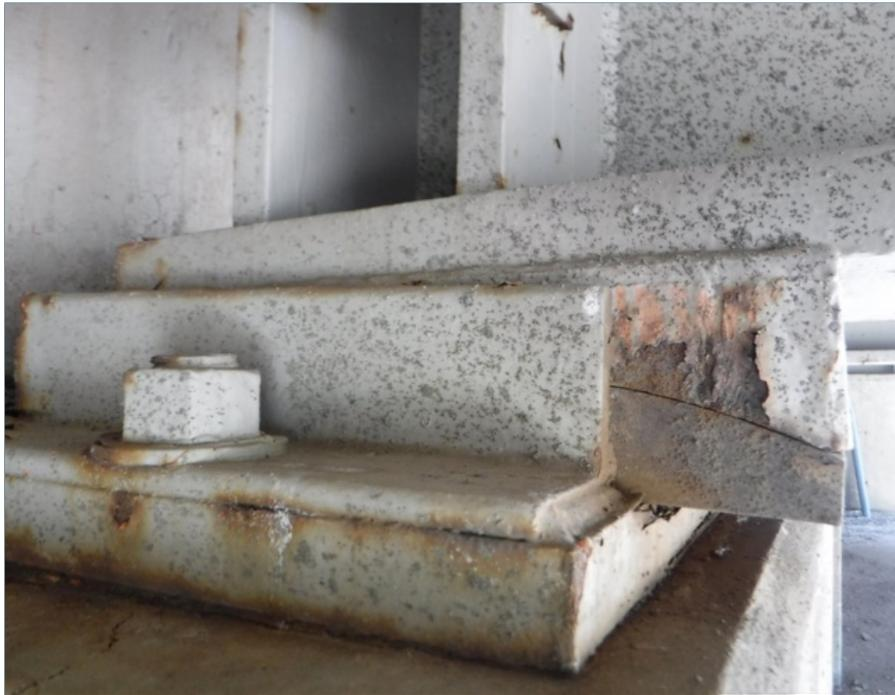
*Figure 2.3-30. Cylindrical bronze bearing (UT)*
