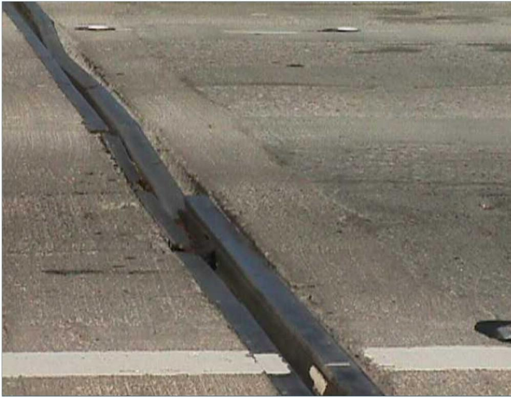
**Figure 2.4-30. Mechanically bonded strip seal failure: Chino Creek, CA**
