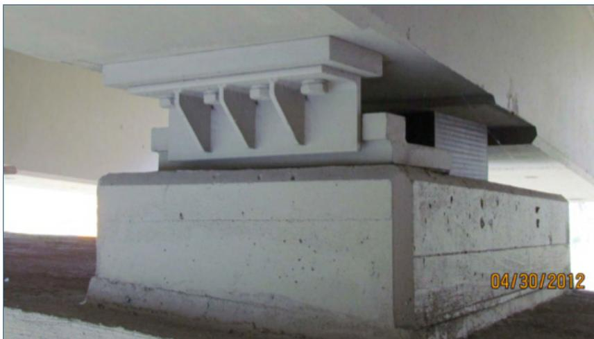
*Figure 2.3-34. External bracket for steel reinforced elastomeric bearing (PA)*
