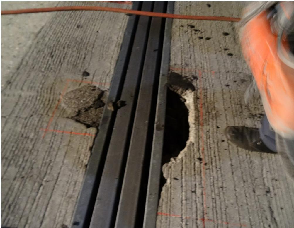
*Figure 2.4-45. Modular joint failure (CA)*
