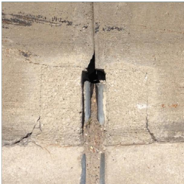
*Figure 2.4-17. No joint in barrier (MI)*
