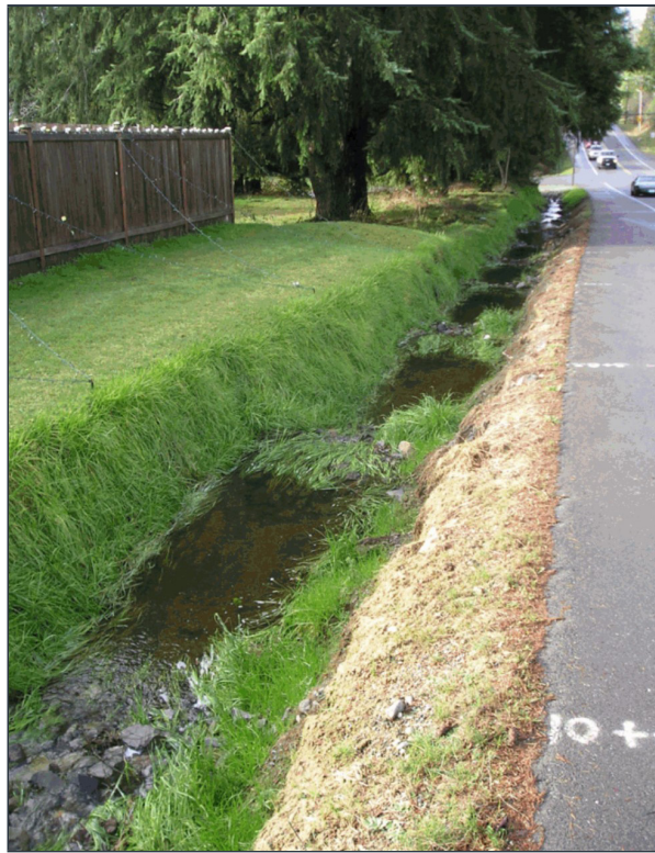
Figure 2-15 King County constructed ditch
