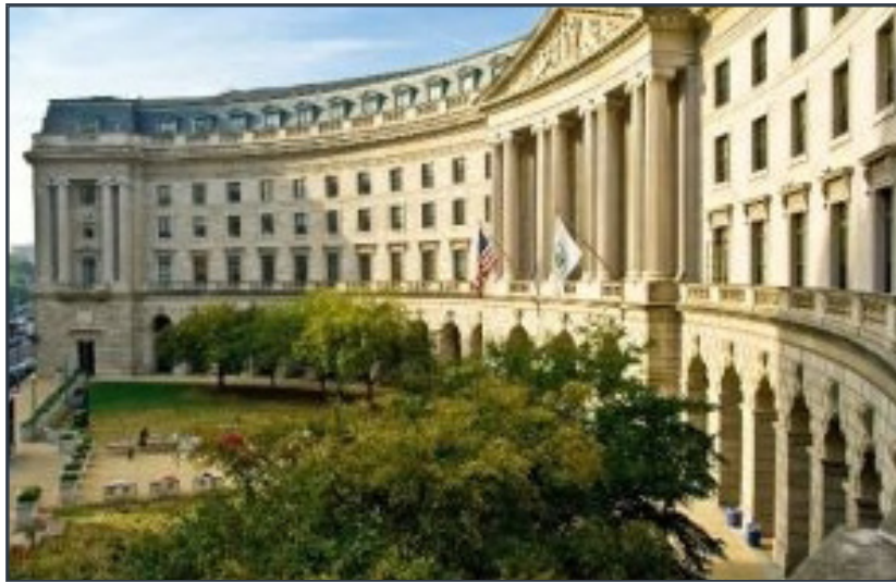
Figure 1-3 Federal buildings, representation of the federal GI Collaborative
