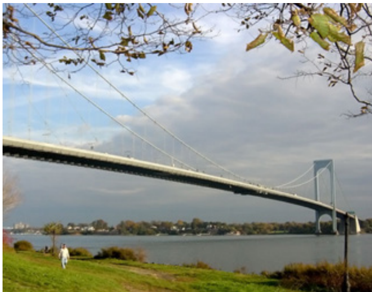
Figure 3-51 The aerodynamic characteristics of the Bronx-Whitestone Bridge were improved with the addition of FRP wind fairings.
