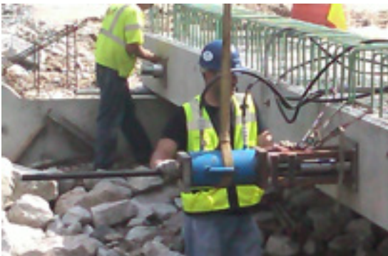
Figure 3-9 Hydraulic jacks apply stress to transverse CFRP PT strands
