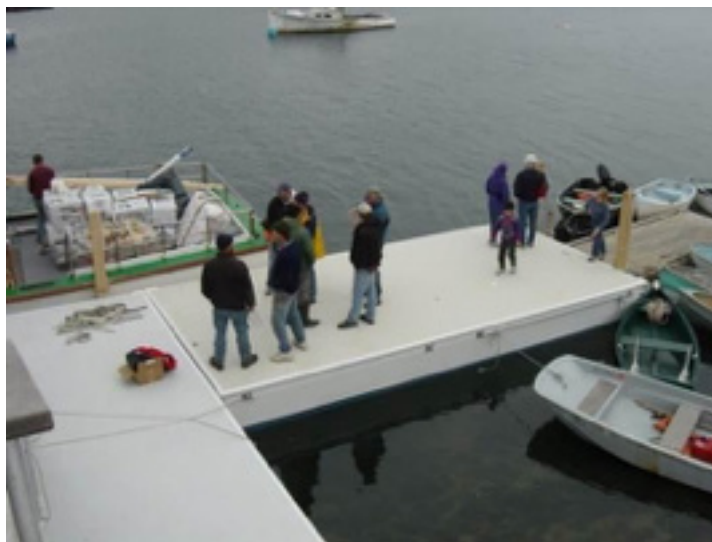
Figure 3-45 FRP floating docks, called floats, outperform timber.
