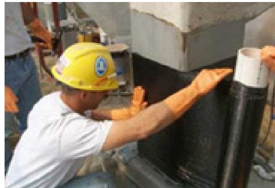
Figure 2-18 Wrapping a square concrete column with CFRP after rounding sharp corners
