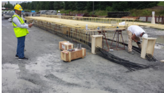
Figure 3-7 Reinforcement and CFRP P/S strands
