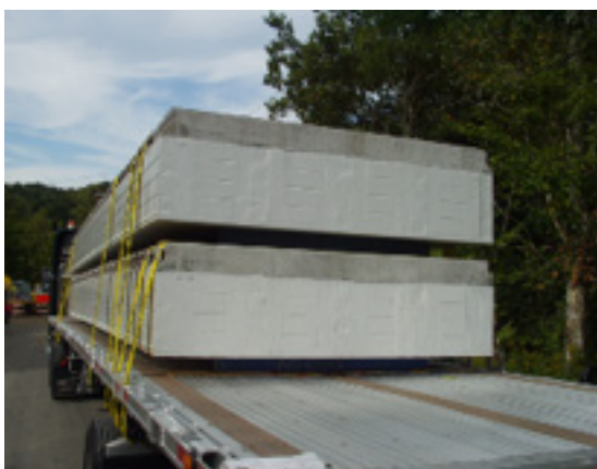
Figure 3-15 FRP/concrete hybrid panels (two of four required for the New Oregon Road bridge)
