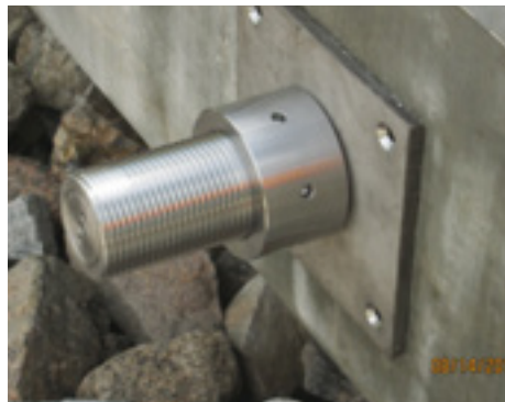
Figure 3-10 Final appearance of transverse PT strand
