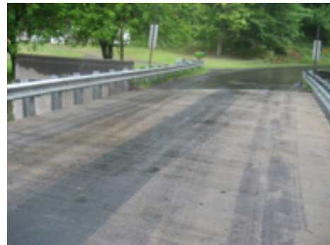
Figure 3-29 FRP deck topped with polymer concrete, subjected to heavy coal trucks
