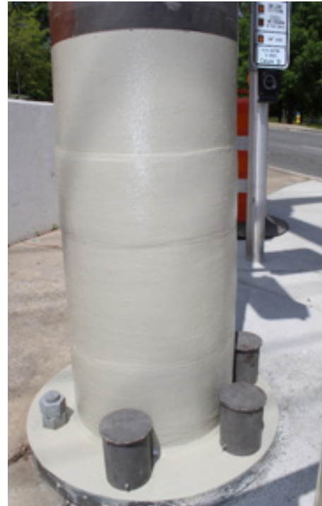
Figure 2-38 Completed pole repair
