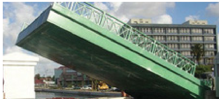
Figure 3-14 A movable bridge fabricated of FRP
