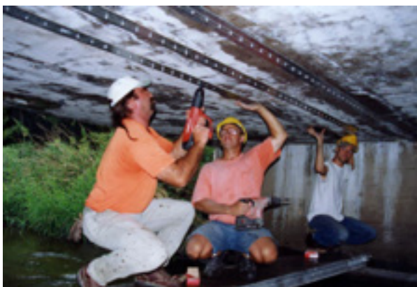
Figure 2-27 Mechanically fastened FRP strips
