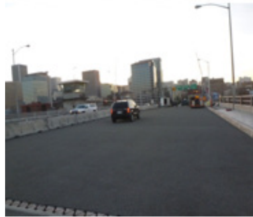
Figure 3-26 FRP on the Morrison Bridge in Portland, Oregon
