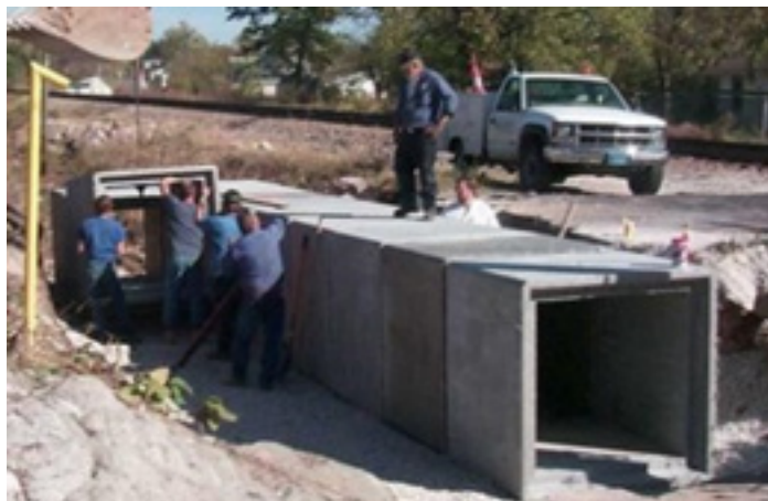
Figure 3-53 A small box culvert
