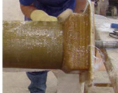
Figure 3-35 Fabrication of an FRP pipe and scupper
