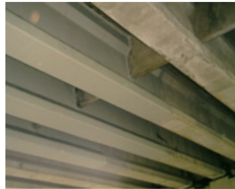
Figure 2-7 Finished repair, after applying UV radiation protective coating
