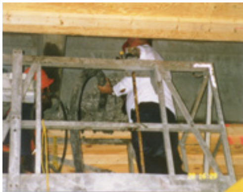
Figure 2-4 Placing concrete to restore the concrete section
