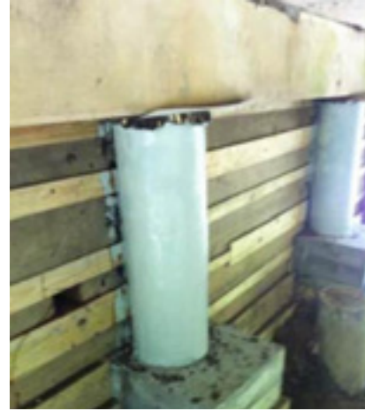
Figure 2-46 3FRP-wrapped timber piles
