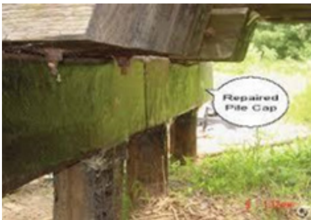
Figure 2-43 FRP-repaired pile cap
