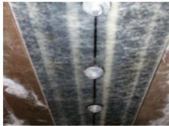
Figure 2-28 Mechanically fastened FRP strip
