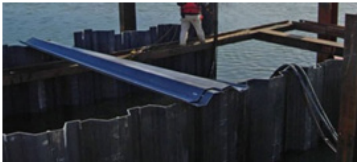
Figure 349 FRP sheeting is damage and corrosion resistant
