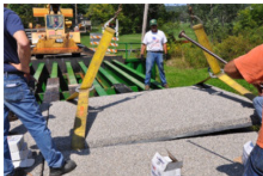
Figure 3-28 FRP deck panels with integral wearing surface
