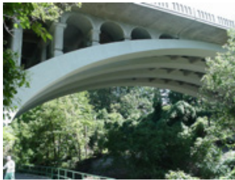
Figure 4-1 A historic concrete arch that was rehabilitated with FRP
