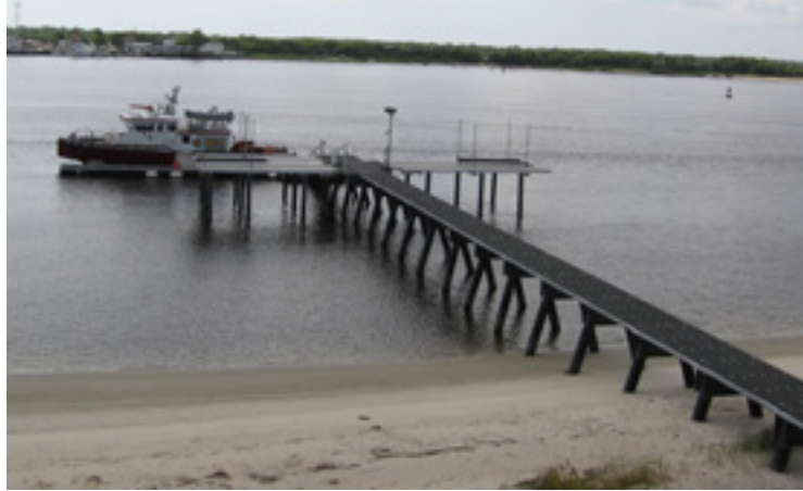
Figure 3-46 An FRP fireboat pier in Florida
