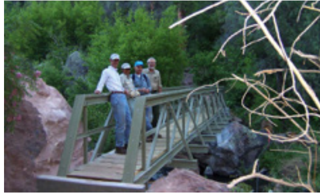
Figure 3-31 A typical FRP trail bridge, easily transported and assembled in remote locations
