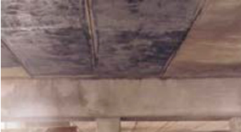
Figure 2-13 Underside of box beams after repair with bonded CFRP
