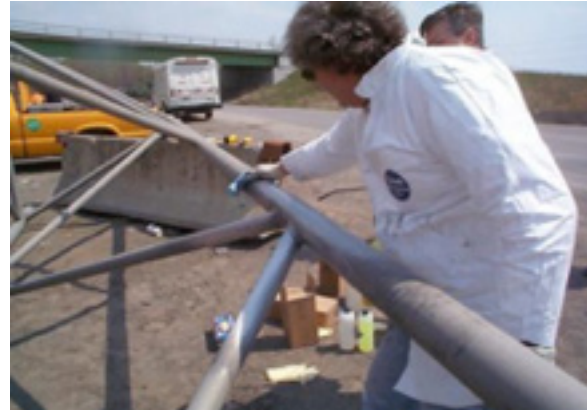
Figure 2-40 Meticulous cleaning (i.e., acid etching) is needed for an FRP repair.
