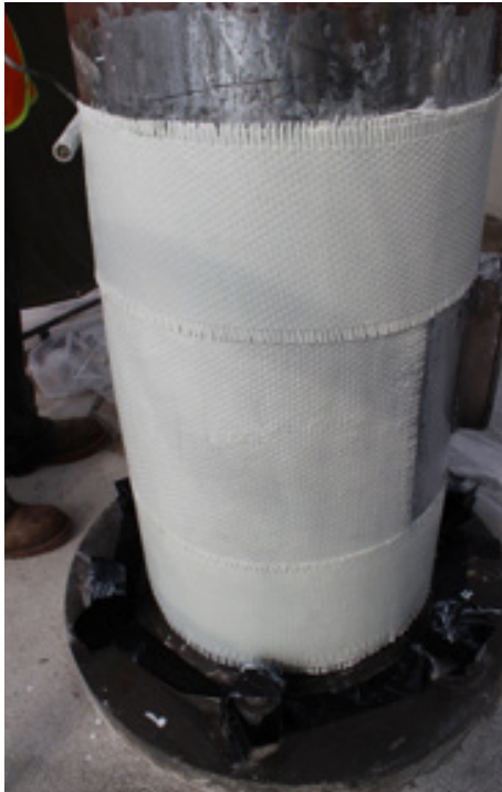
Figure 2-37 GFRP wrap being applied
