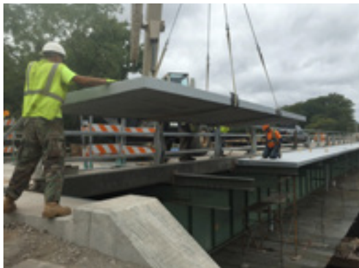
Figure 3-32 Installation of a lightweight sidewalk panel
