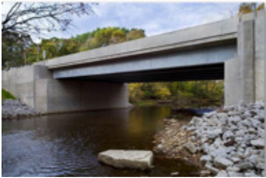
Figure 3-17 High Road over Long Run Creek in Illinois
