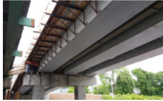
Figure 3-18 Route 49 over Ottery Creek Overflow in Missouri
