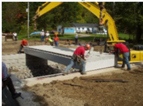
Figure 3-16 Placement of a prefabricated hybrid panel (see Fig 3-15)
