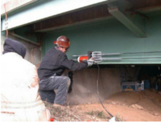
Figure 2-30 300 ksi CFRP rods (3/8") being jacked to post-tension a steel girder
