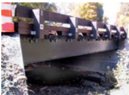
Figure 3-13 Corrosion-resistant FRP beams (double web)
