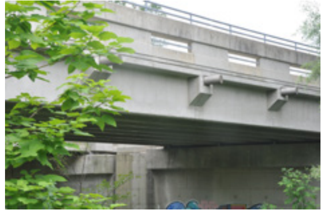
Figure 2-26 Transverse CFRP post-tensioning of concrete beams
