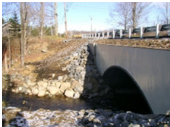
Figure 3-21 The completed arch structure
