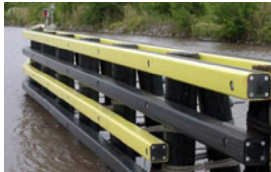
Figure 3-42 Wales fabricated with GFRP bars encased in resins
