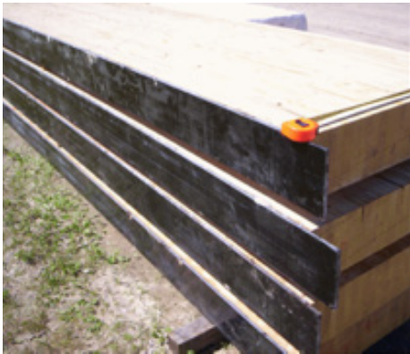
Figure 3-22 Glu-lam beam with FRP plate bonded to the bottom
