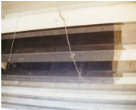
Figure 2-6 CFRP bonded to the repaired concrete section
