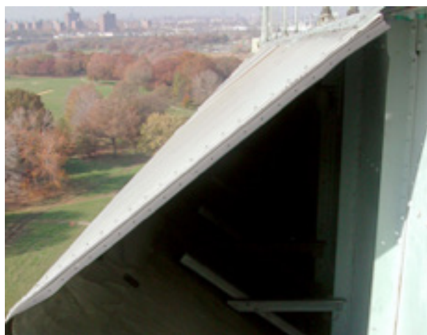
Figure 3-52 The wedge shaped wind fairing used on the Bronx-Whitestone Bridge, which is a twin of the ill-fated Tacoma-Narrows Bridge.
