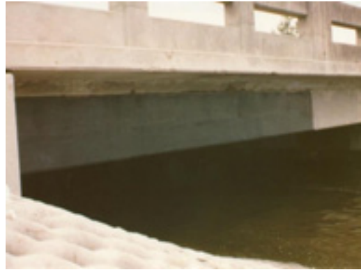
Figure 2-9 Bonded CFRP repair of beams shown at left
