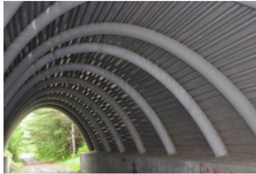
Figure 3-19 An underpass for recreational vehicles constructed with concrete-filled FRP tubes
