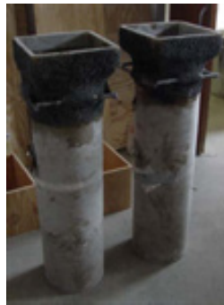
Figure 3-36 Combined FRP scupper and drain pipe
