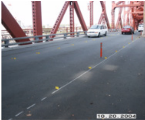
Figure 3-25 FRP on the Broadway Bridge in Portland, Oregon
