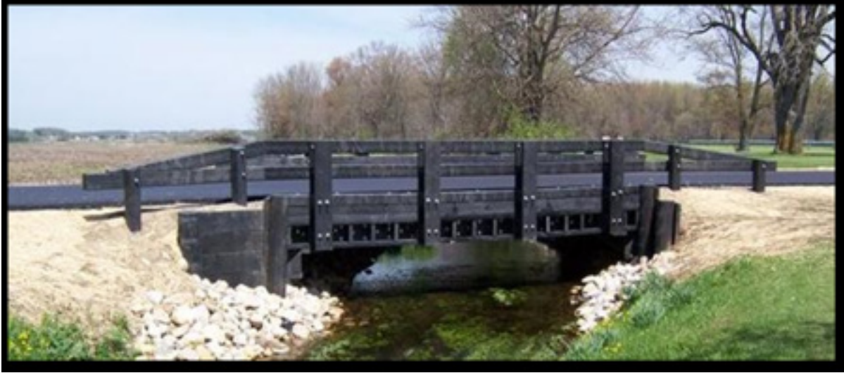
Figure K3 Completed thermoplastic bridge in Ohio, opened in 2011
