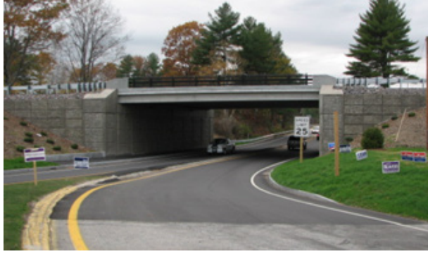
Figure 3-8 Completed bridge in Kittery, Maine, with carbon P/S
