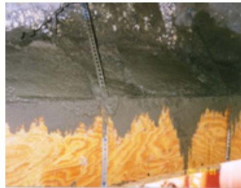
Figure 2-5 Restored section, prior to removing the forms
