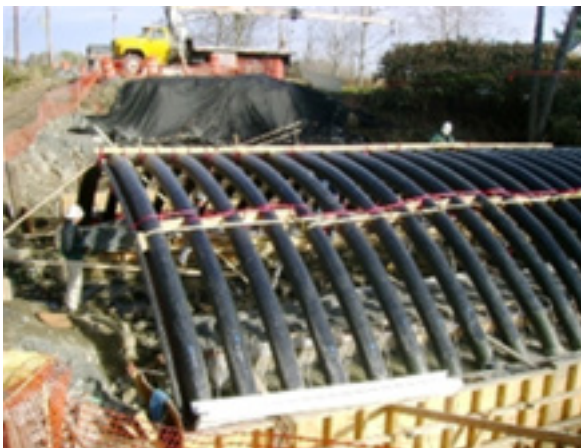
Figure 3-20 FRP tube arches erected
