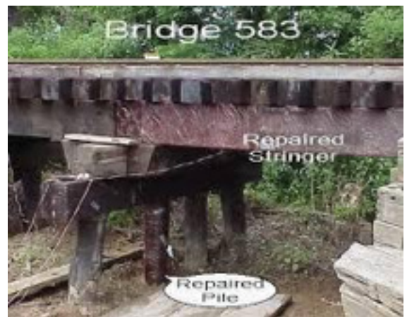
Figure 2-44 FRP-repaired timber piles and stringers
