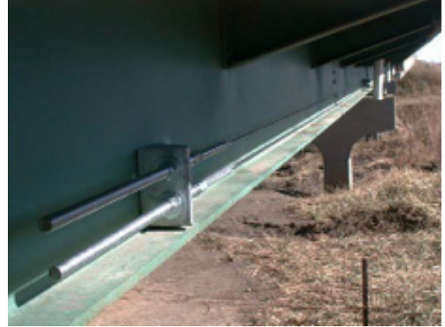
Figure 2-31 Post-tensioning with CFRP
