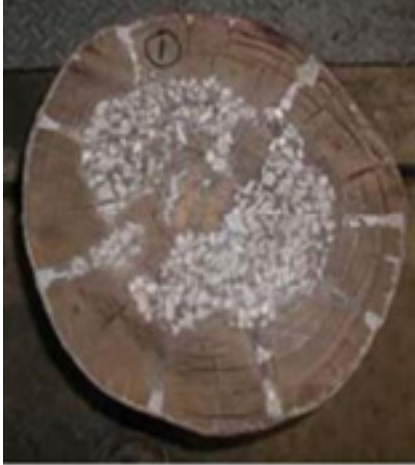
Figure 2-45 Timber pile impregnated with resin to fill voids
