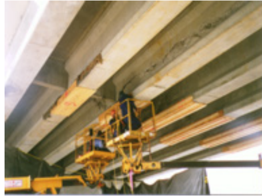
Figure 2-3 Formwork preparation for replacing the damaged concrete
