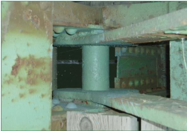
**Figure 3-2** *Pack rust between eyebolt head and adjacent gusset plate before ultra-high-pressure washing*
