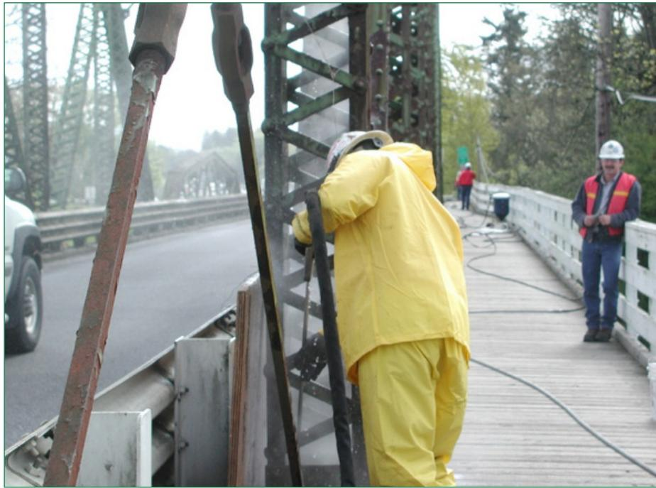
**Figure 3-1** *Ultra-high-pressure washing to remove pack rust on Willamette River Bridge in Corvallis, OR*
