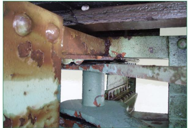
**Figure 3-3** *Pack rust removed using ultra-high-pressure washing*
