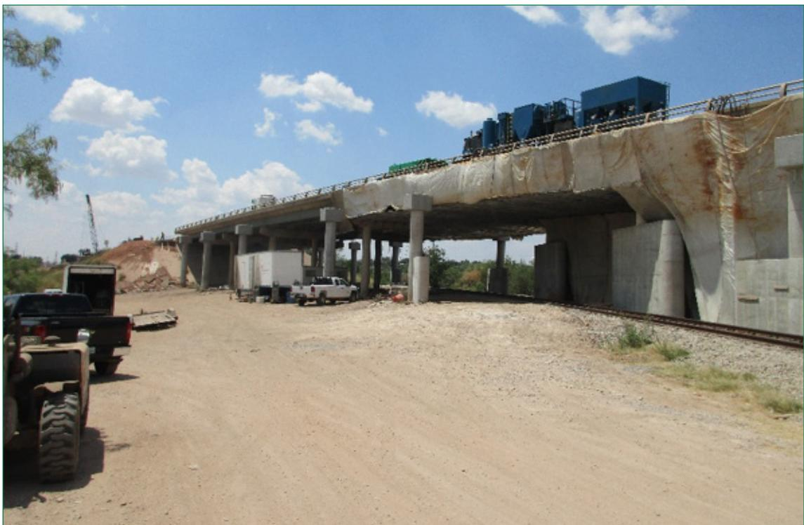
**Figure 2-2**     **Containment for US 67 over Texas Pacifico Railroad in Ballinger, TX**
