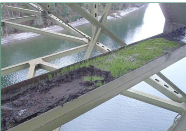
**Figure 3-4** WSDOT bridge before cleaning
