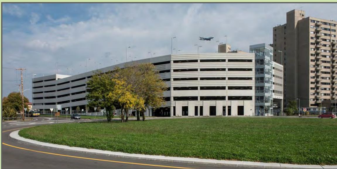
Figure 3.5 Garage at Wonderland Transit Station, Revere, Massachusetts
