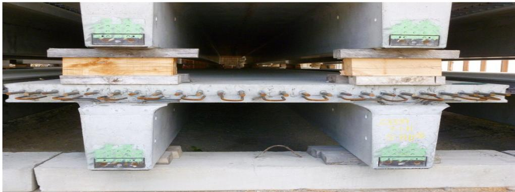
*Figure 2.53 NEXT double-T girder used in Massachusetts*
