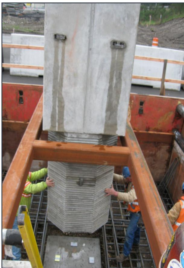
Figure 2.15 Precast column to CIP footing connection in Washington State
