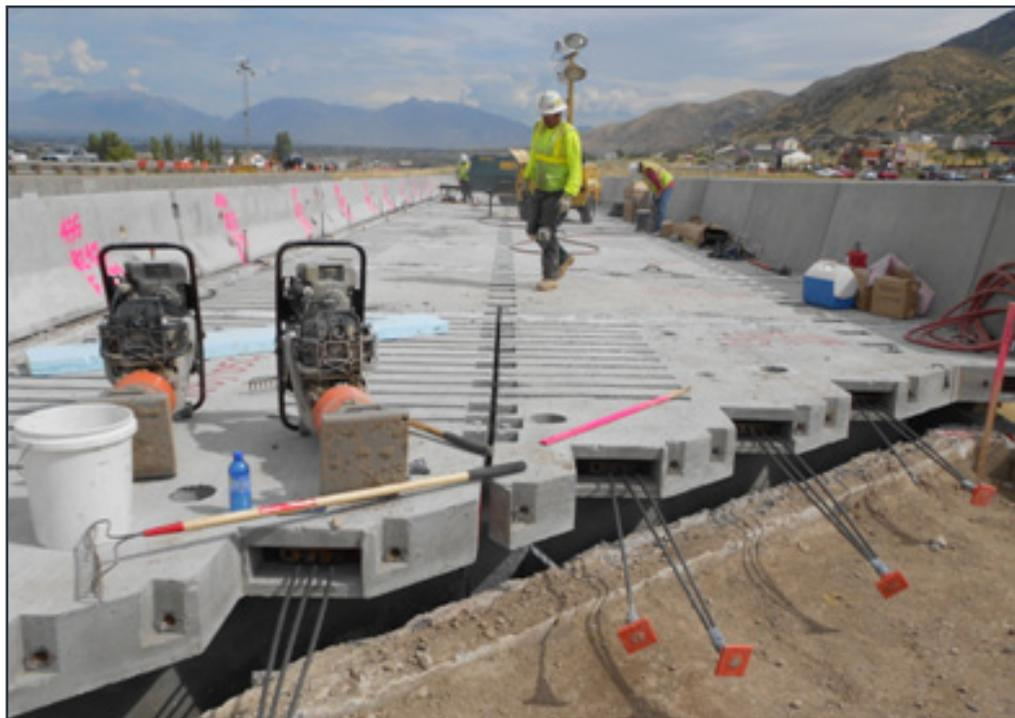
Figure 2.14 Deck post-tensioning in Utah
