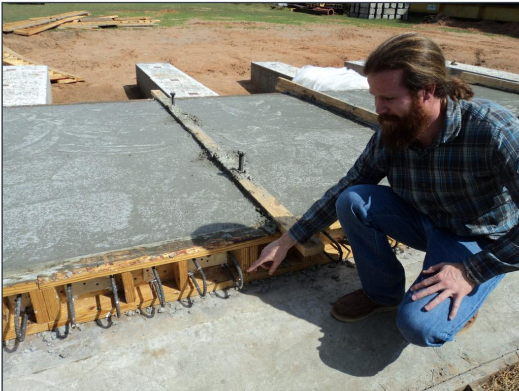
*Figure 2.12 Full-depth precast deck panel connection*
