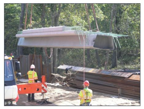
Figure 2.54 Folded plate girder bridge in Massachusetts
