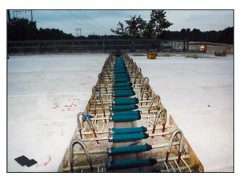
Figure 2.21 Grouted coupler as continuity splice over pier in Massachusetts
