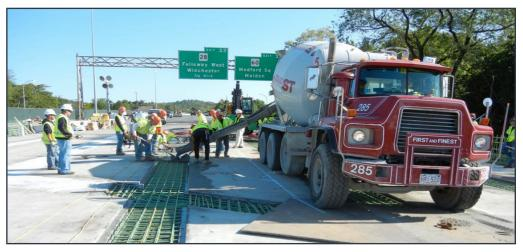
Figure 2.13 Deck closure pour construction in Massachusetts Fast 14
