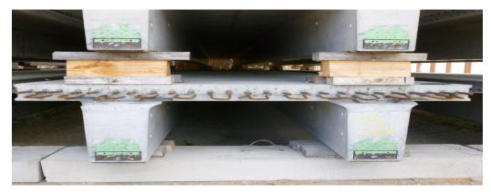
Figure 2.53 NEXT double-T girder used in Massachusetts
