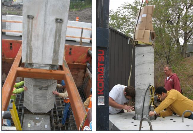
Figure 2.15 Precast column to CIP footing connection in Washington State
