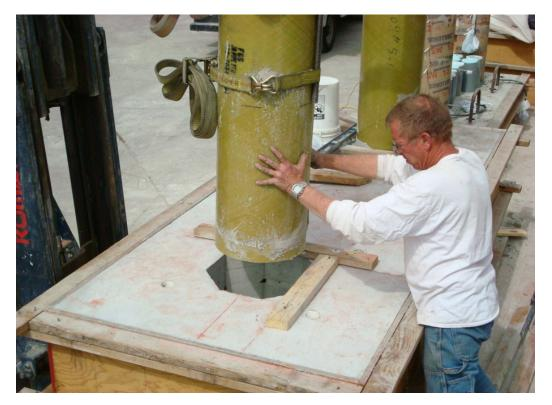
Figure 2.48 Precast concrete-filled FRP tube column at UNR
