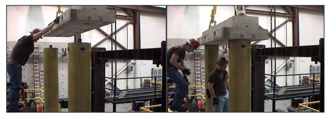
Figure 2.51 Lowering a precast cap beam onto steel pipe pin connections of a concretefilled FRP tube pier at UNR
