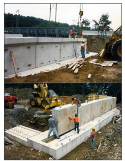
Figure 2.19 Precast abutment wall andfootings with grouted coupler connections in Massachusetts
