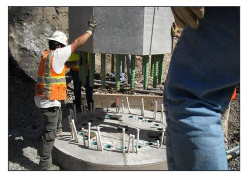
*Figure 2.22 Precast column connection to pile shaft with embedded grouted coupler in Utah*
