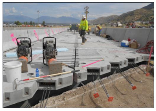
Figure 2.14 Deck post-tensioning in Utah
