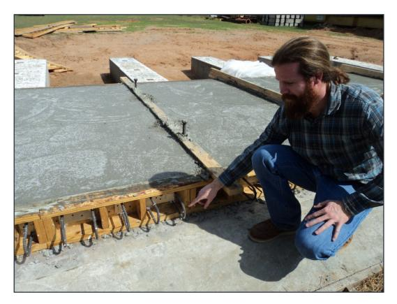
Figure 2.12 Full-depth precast deck panel connection
