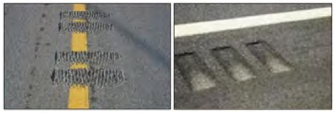
Figure 3.1 Examples of CLRS (left) and SRS (right)
