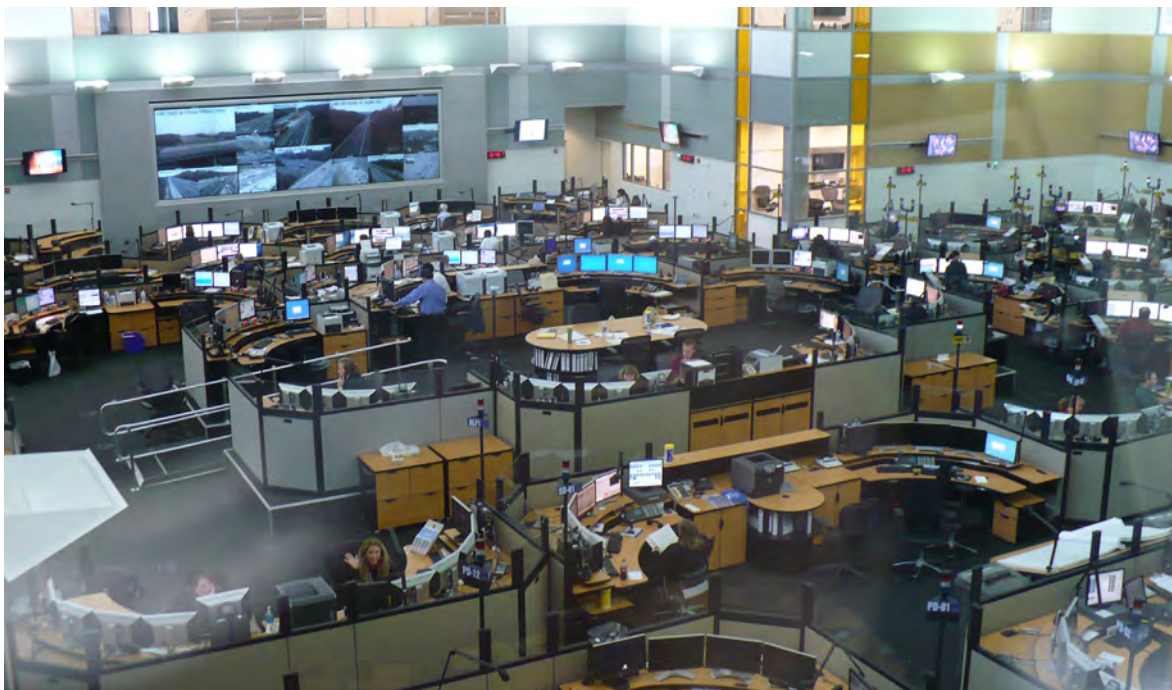
Figure 2.3 View of the McConnell PSTOC from the raised supervisor station
