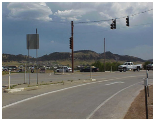
Figure 3.6 Temporary traffic signals in Sturgis, South Dakota (photo courtesy of Doug Kinniburgh)
