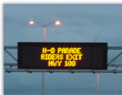
Figure 3.9 Permanent variable message signs alert riders to expected destinations
