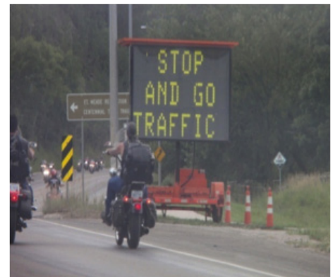
Figure 2.1 Advance notice of changed conditions. This message alternates with “BE PREPARED TO STOP” (photo courtesy of Doug Kinniburgh)
