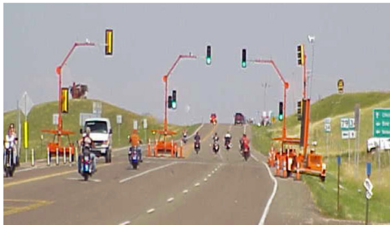
Figure 2.3 Portable traffic signals in Sturgis, South Dakota (photo courtesy of Doug Kinniburgh)
