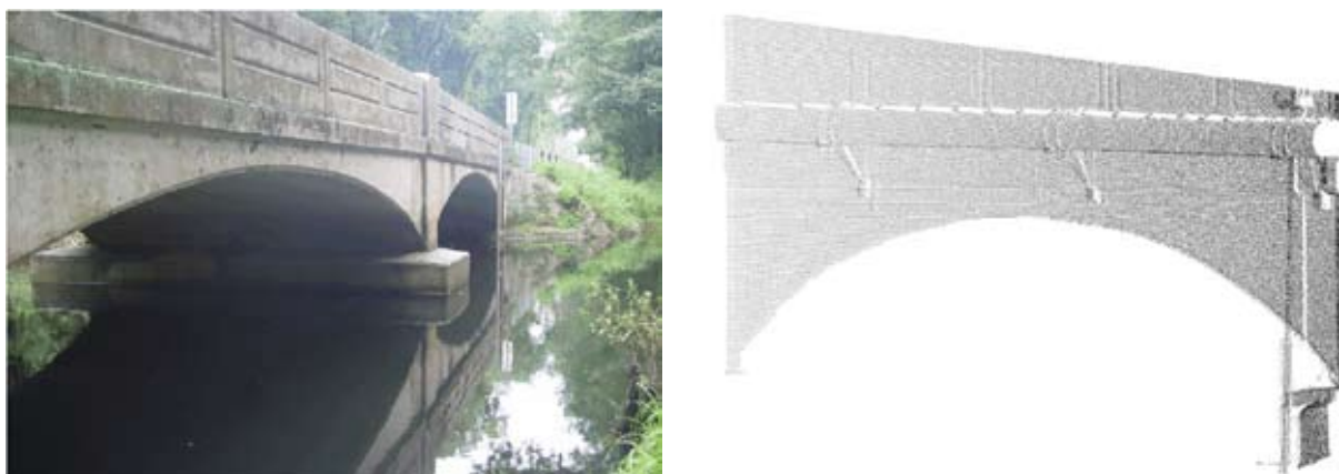
Figure 6.4 Florida bridge and surface scan 22
