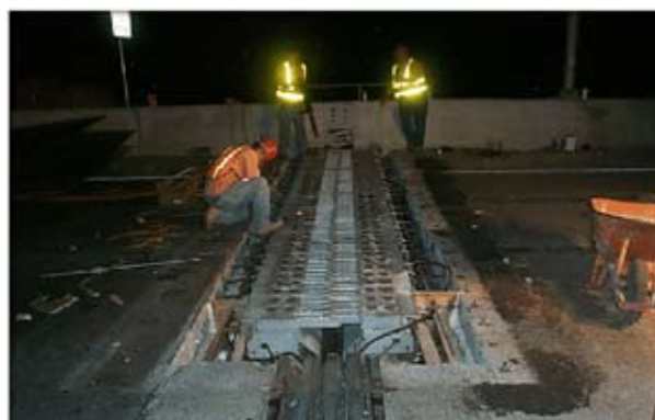
Figure 6.2 Florida joint replacement 15
