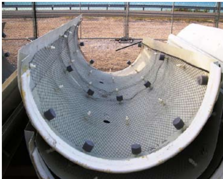
Figure 6.5 Florida mesh in pile jacket form 23
