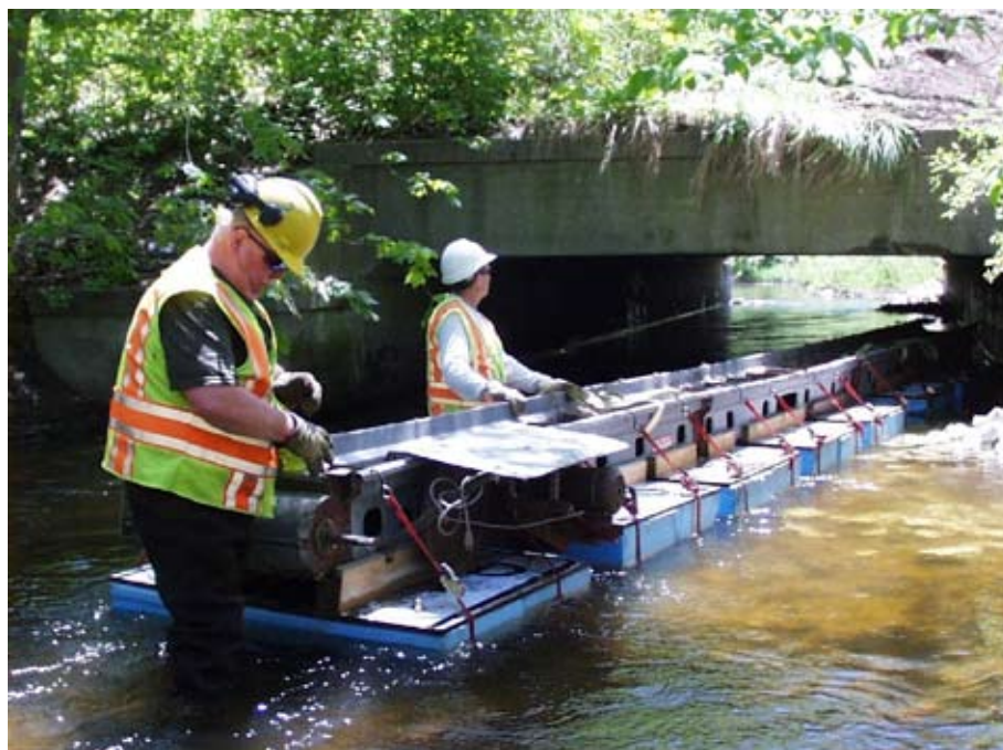
Figure 8.3 Michigan Southwest region's floating conveyor for rip rap 34
