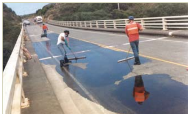
Figure 2.3 Deck treatment with HMWM 4
