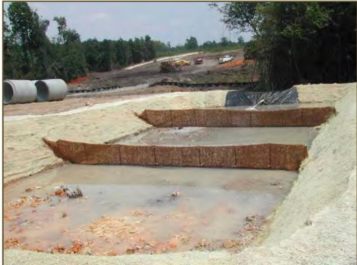
**Figure 4.19** Sediment basin with baffles on a NCDOT project
