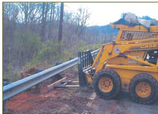
**Figure 5.3** NCDOT sheet flow maintenance tool
