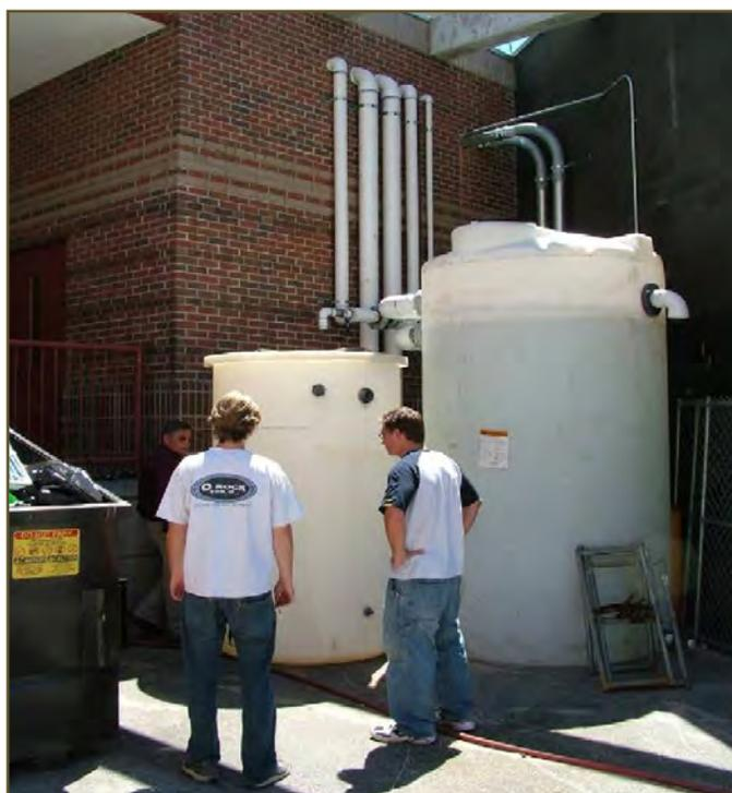
**Figure 4.15** *Stormwater harvesting cistern at UCF*
