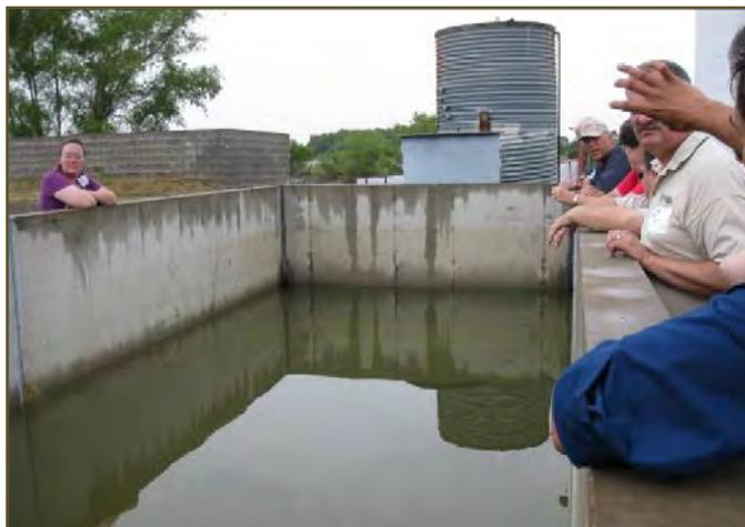
**Figure 4.14** *Nonproprietary stormwater vault prototype at TTI*
