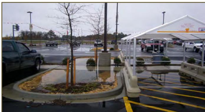
**Figure 4.8** *Slow-draining infiltration area*
