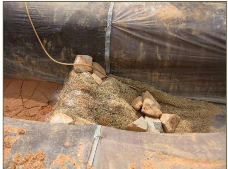
**Figure 4.18** Rock check dam with PAM visible
