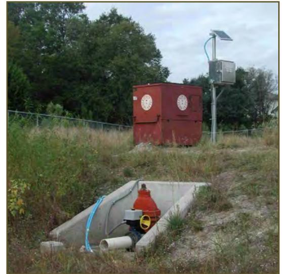
**Figure 4.11** *Batch detention automated valve and PLC*
