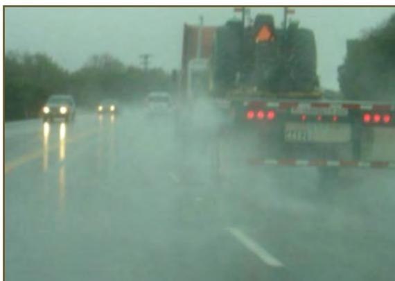
**Figure 4.12** *Dense graded asphalt during a rainstorm*
