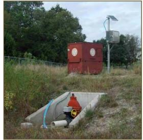
Figure 4.11 Batch detention automated valve and PLC
