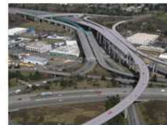
Nalley Valley Viaduct after the new westbound structure is completed.
