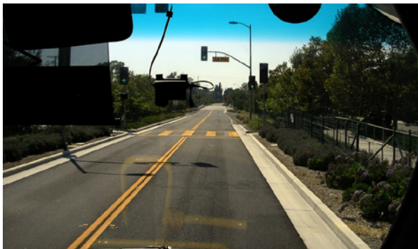
Lessons learned from the Right-of-Way scan helped speed construction on Connecticut DOT's Busway project.
