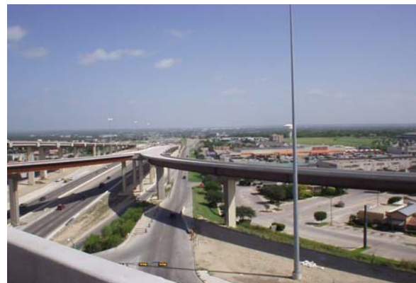
Interchange at SH 45 and I-35.
