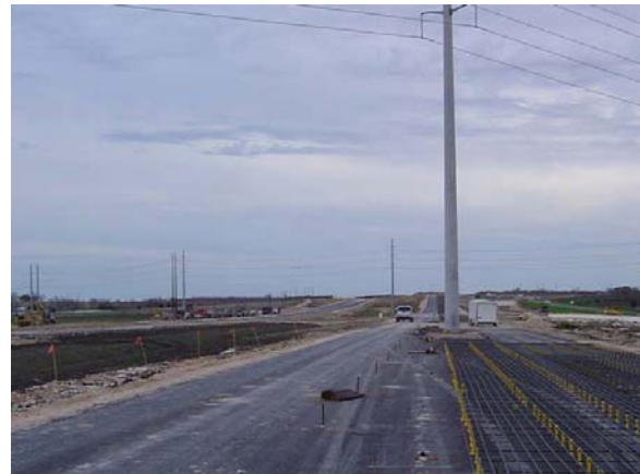
In some cases, utility adjustments were still being negotiated and completed while construction was underway, as was the case with this utility pole that needed to be moved from the highway median.
