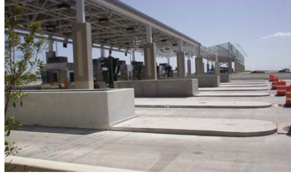
A 22-lane toll plaza on Loop 1 in Austin. This facility will allow high-speed toll collection with the use of TxPass electronic toll collection.
