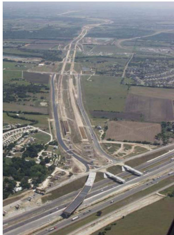
SH 130 looking southeast from its interchange with I-35.
