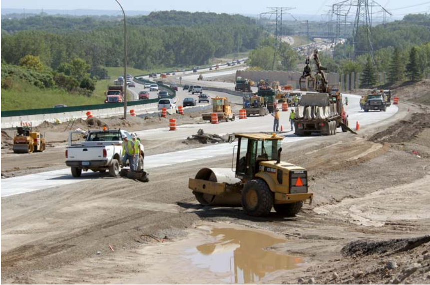
I-494 Phase 2 reconstruction in Minneapolis' western suburbs.
