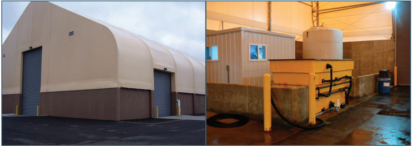
Figure 2-39. This soft-top building stores both solid and liquid chemicals and has its own brine-making facility. Trucks drive through so all loading is done inside. (INDOT)
