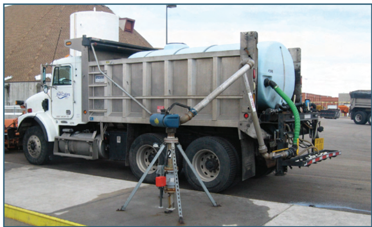
Figure 2-38. Trucks are loaded with liquids using a system similar to a fuel-dispensing station with the ability to keep track of which agency draws material for which truck. Solid chemicals that are loaded are automatically weighed. Both liquids and solids are dispensed to multiple agencies. (City of Ft. Collins, CO)
