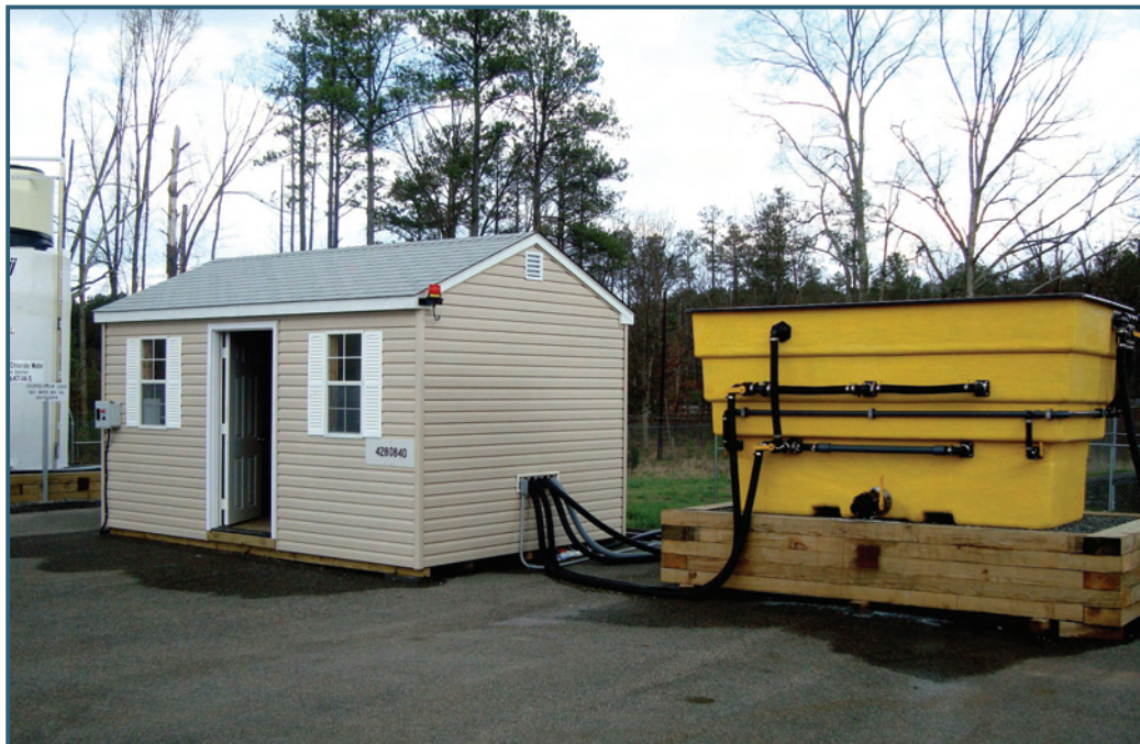
Figure 2-43. Brine storage and brine makers must have protection from spills or leaks. Note the wood wall around base of this salt brine maker. (VDOT)
