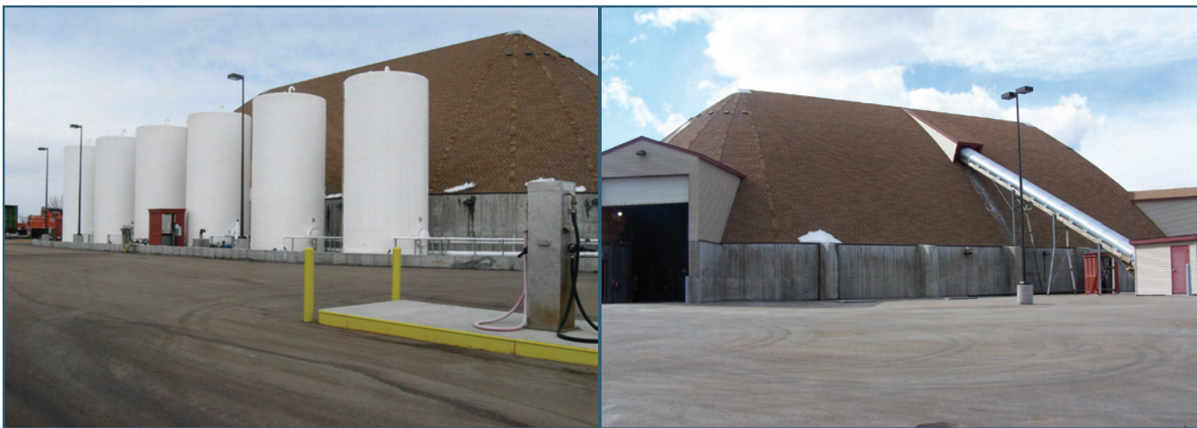
Figure 2-37. Solid chemical storage building designed for stockpiling via conveyor and inside loading of trucks during winter events; liquid storage is alongside. (City of Fort Collins, CO)
