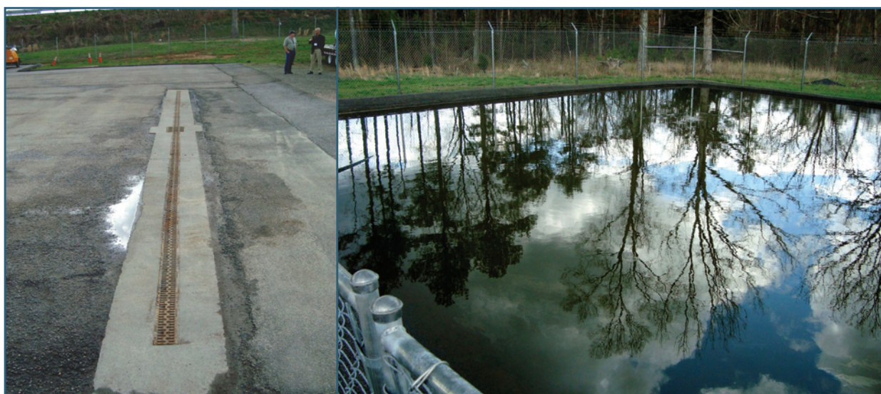
Figure 2-41. To be environmentally friendly, chemical storage and loading areas need to be designed to prevent runoff from leaving the property. Collection drains and collection ponds are a means to do that. (VDOT)
