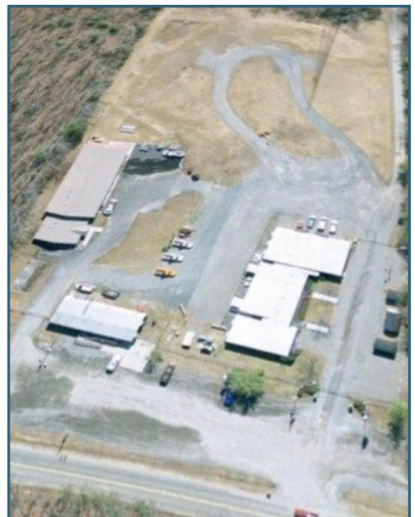
Figure 2-47. VDOT Maintenance Training Academy (VDOT)
