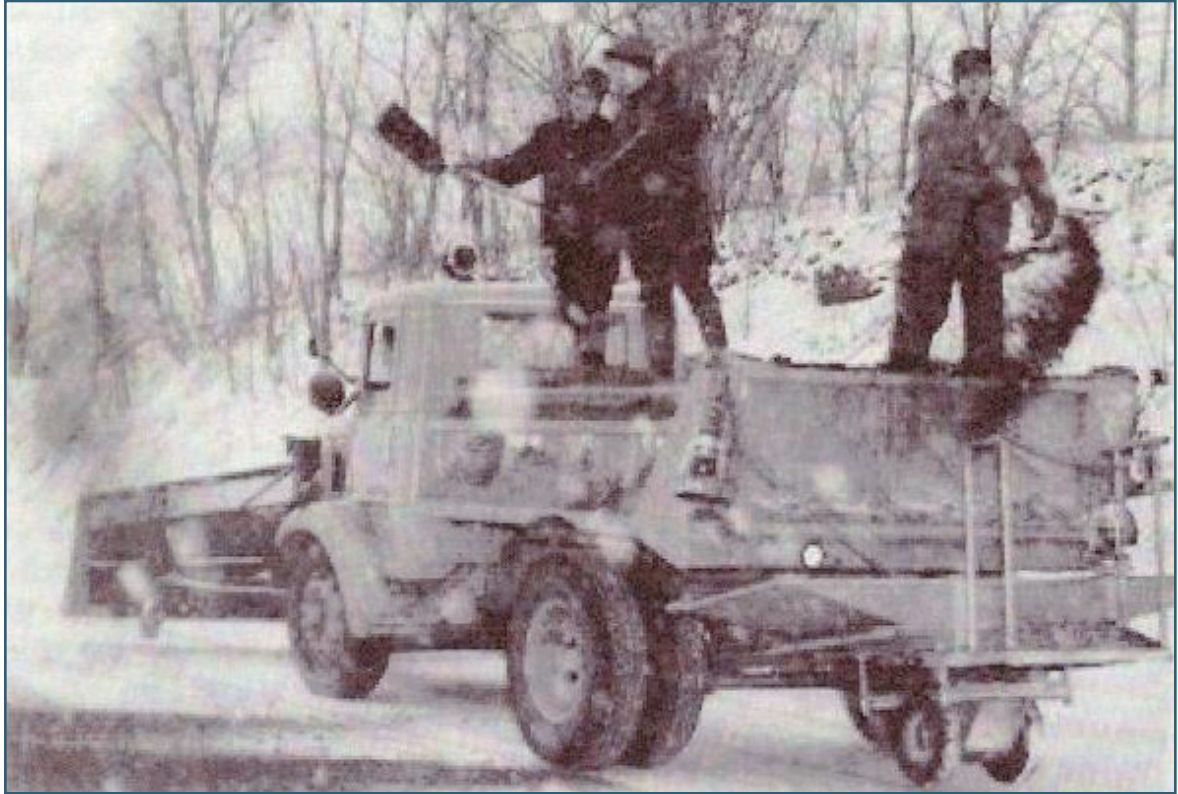
Figure 1-2. Here is an old photo of the original style of spreading sand or cinders on the Pennsylvania Turnpike in the early 1940s. (PennDOT)
