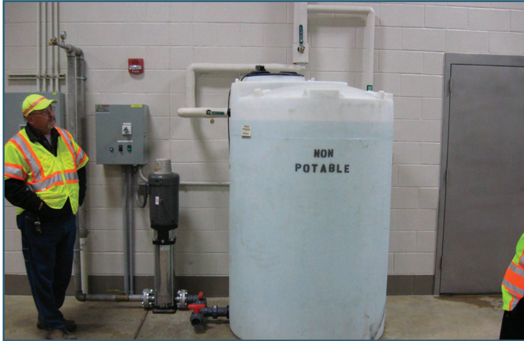
Figure 2-42. Wash water from washing chemical-spreading trucks is contaminated with dissolved salt and needs to be collected and reused, treated or properly disposed of. (INDOT)
