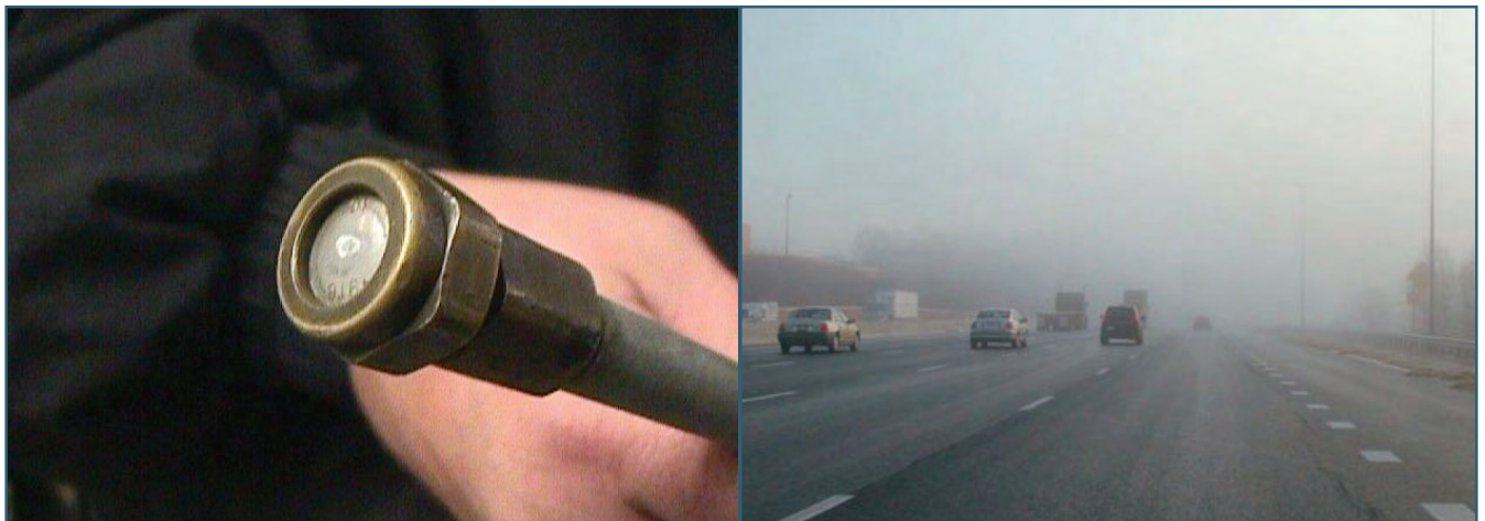
Figure 2-31. Nozzles on the fog dispersal system distribute CO 2 to lift fog away from the travel lane. (UDOT)
